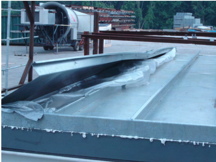
Photo No. 7 Test Specimen #3 – Failure Mode
