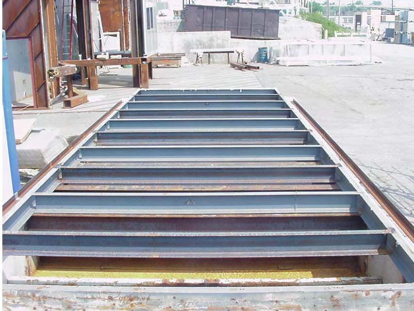
Photo No. 4 Corner Condition – Purlin Spacing
