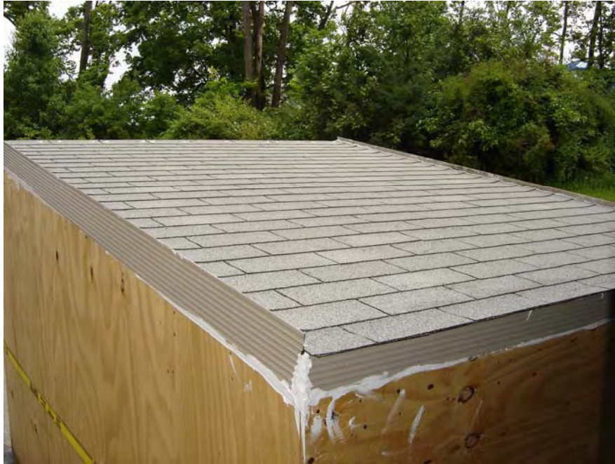
Photo No. 1 Roof System Prior to Test
