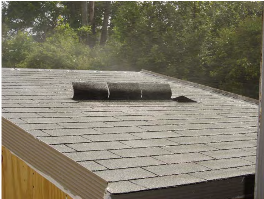
Photo No. 4 Roof System During 90 MPH Phase
