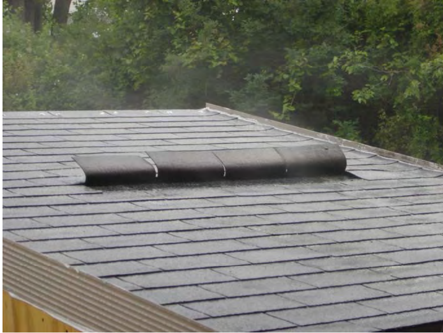
Photo No. 5 Roof System During 110 MPH Phase
