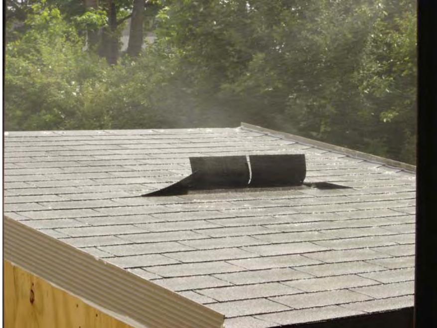
Photo No. 3 Roof System During 70 MPH Phase
