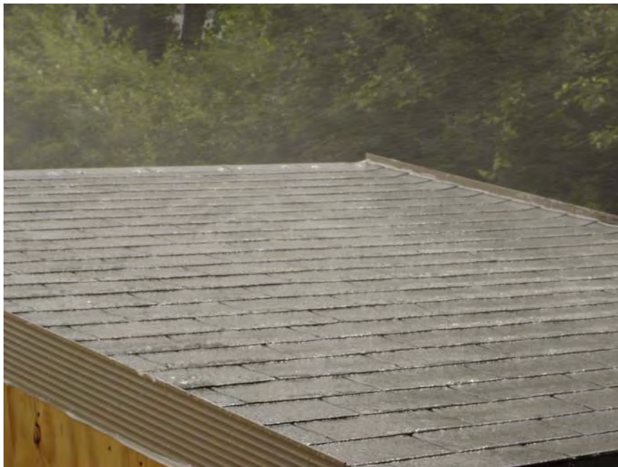
Photo No. 2 Roof System During 35 MPH Phase
