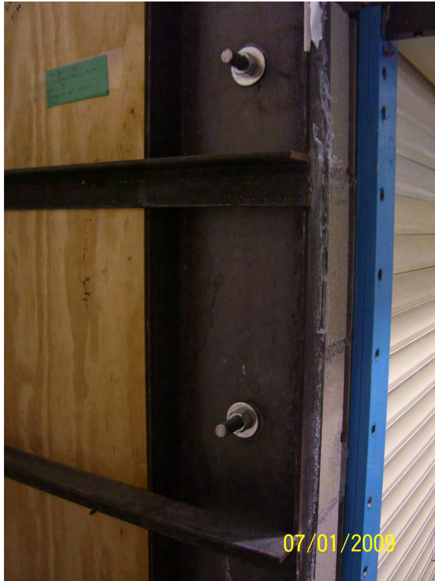
Photo No. 1 Test chamber construction
