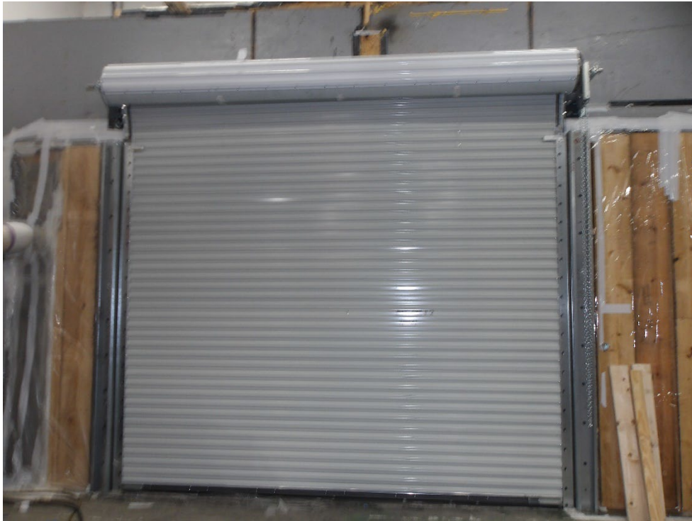
Photo No. 1 Interior of Door, Exterior of Chamber
