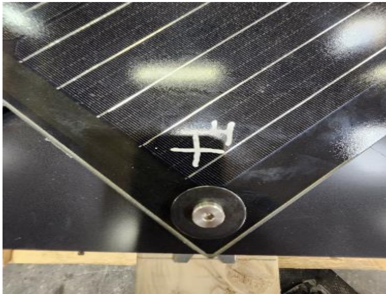
Photo No. 9 Impact Location #4 After Impact
