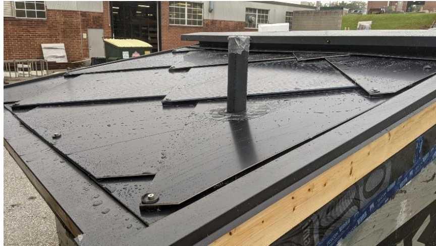
Photo No. 19 Post Test Top Side
