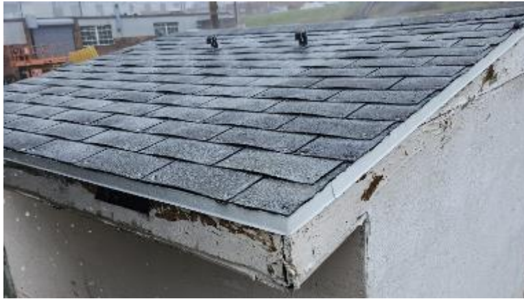
Photo No. 11 Post Test Top Side
