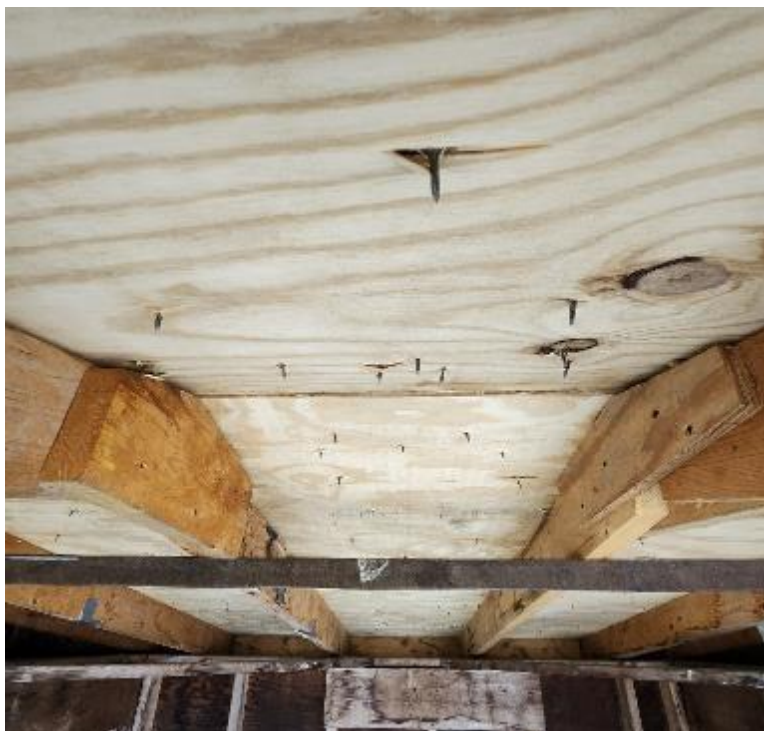
Photo No. 10 110 MPH Underside
