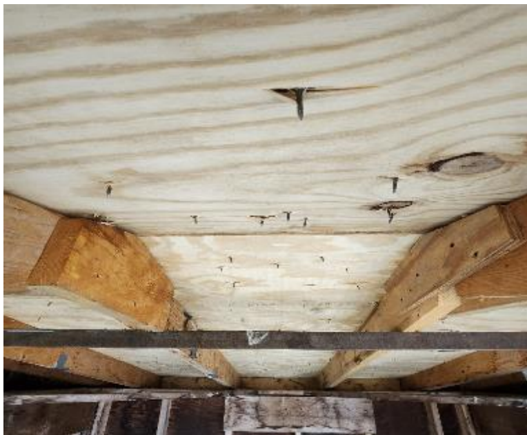
Photo No. 2 Underside Before Testing
