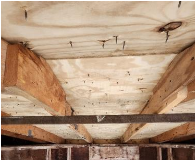
Photo No. 8 90 MPH Underside
