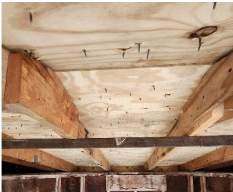
Photo No. 4 35 MPH Underside
