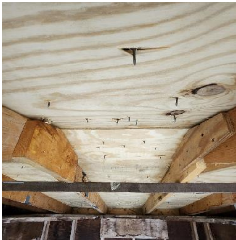
Photo No. 6 70 MPH Underside
