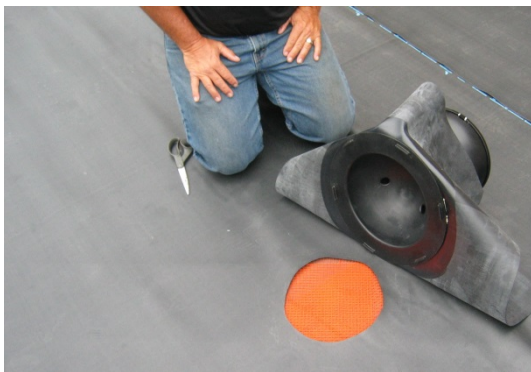
An Opening is Cut in the Roof Membrane for the V2T Vent
