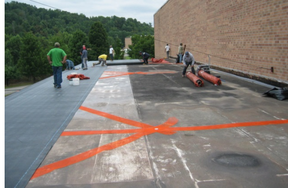
Roof Membrane is Placed Over the Distribution Strips
