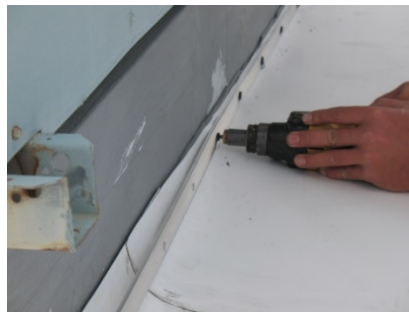
Fasten Termination Bar 6" o.c.
