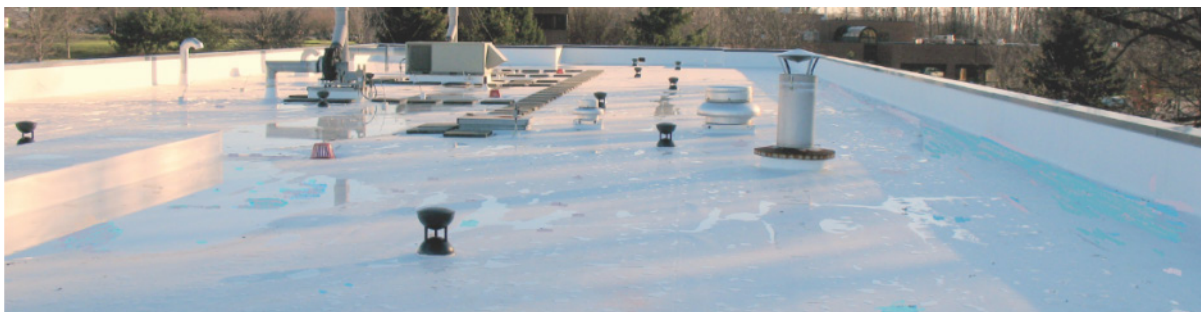
Position of V2T Vents are Staggered to Accommodate Variations in Wind Speed on a Completed Roof Application
