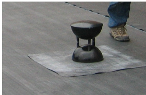
Skirt on the V2T Vent is Adhered Using Double-Sided Butyl Tape to the Roofing Membrane
