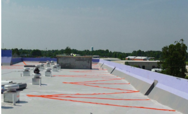
Distribution Strips Connect the Roof Perimeter to the V2T Vents
