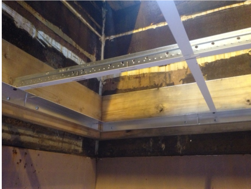
Photo No. 1 Perimeter, Main, and Tee Detail
