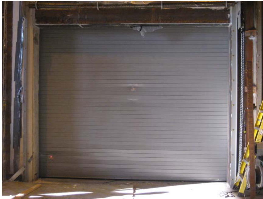
Photo No. 1 12' 4" x 10' Roll-Up Garage Door
