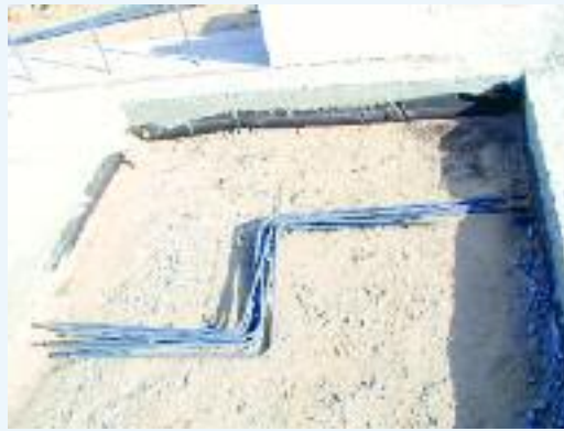
Figure 8.2 – Pre-cut & bent reinforcing steel will increase efficiency
