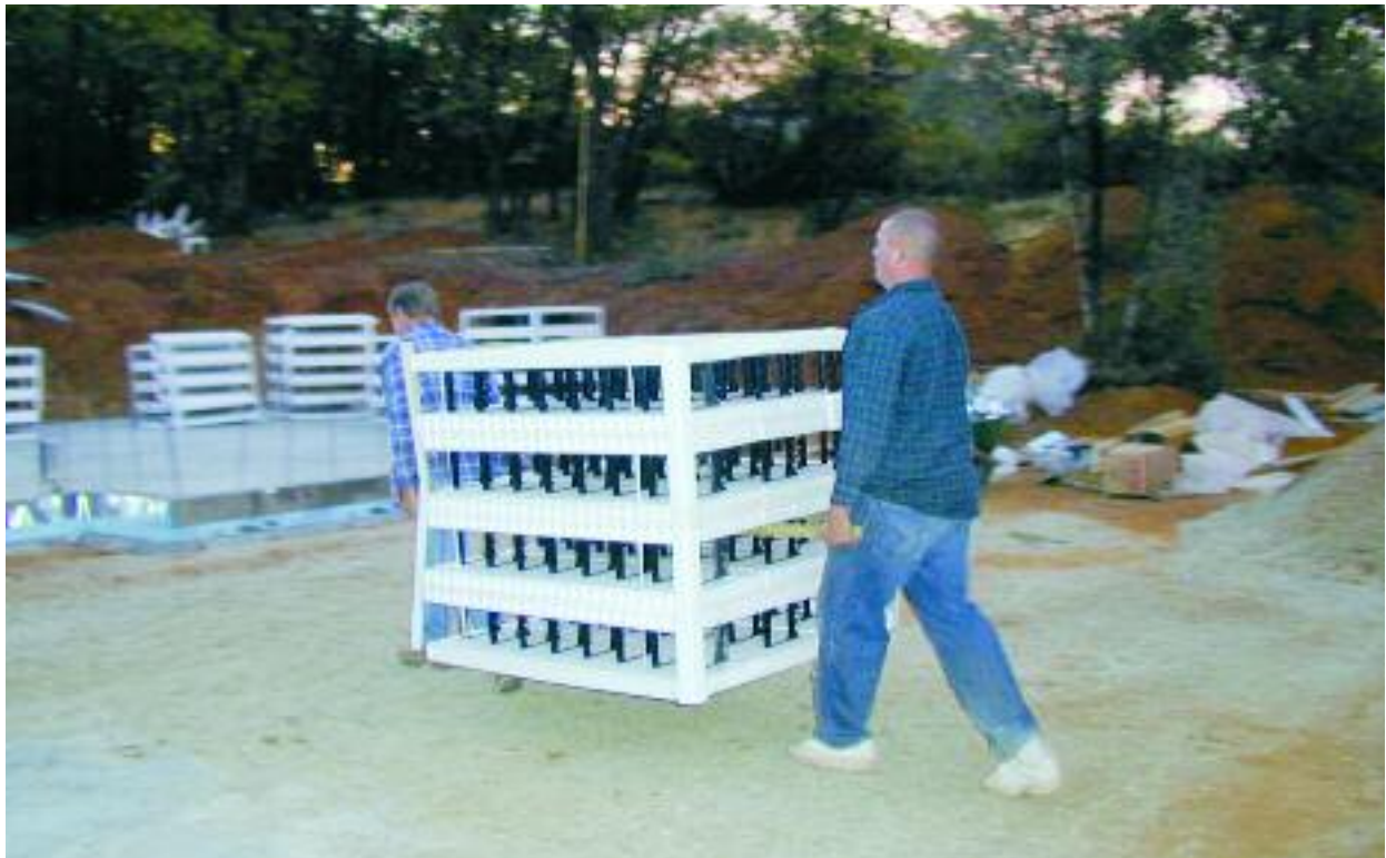
Figure 8.3 – Moving ICF bundles by hand
