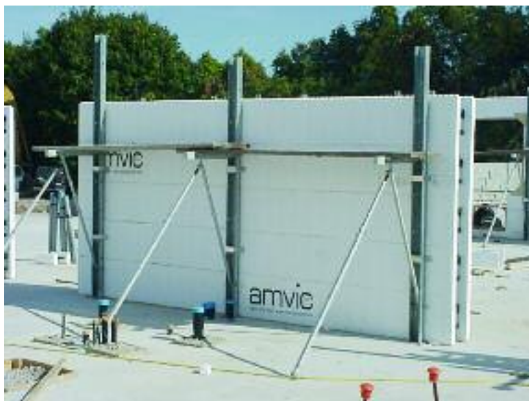
Figure 8.30 –Platform and scaffold planks
