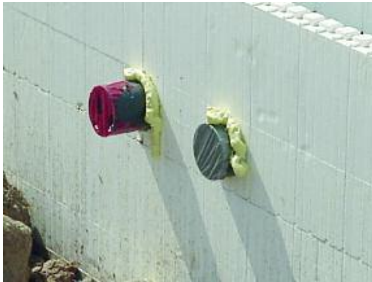
Figure 8.41 – Using PVC pipe for penetration block-outs
