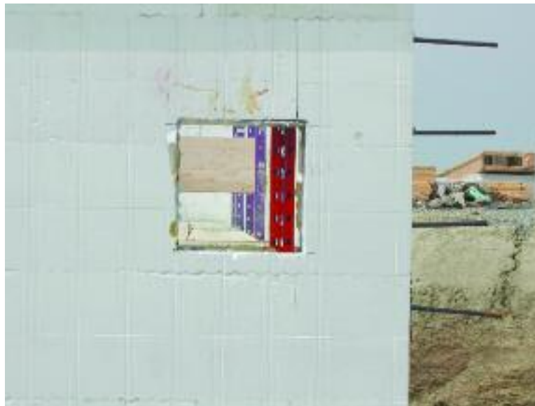
Figure 8.54 – Cut out opening from the inside and outside EPS panels on one side
