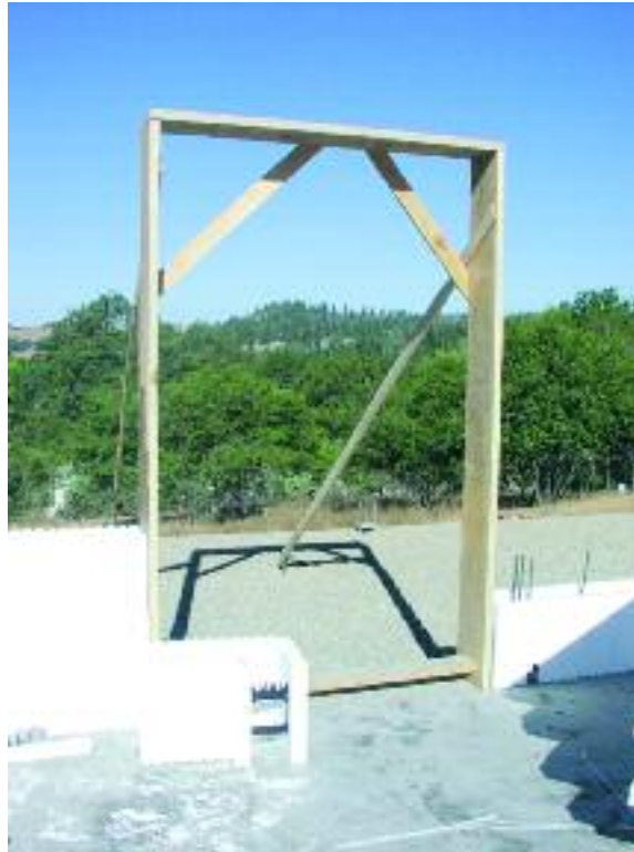
Figure 8.7 – Placing Door Bucks
