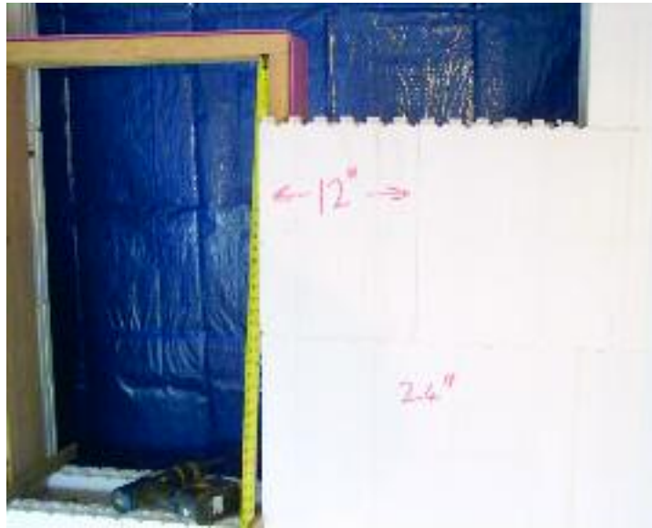
Figure 8.24 – Building courses around window bucks
