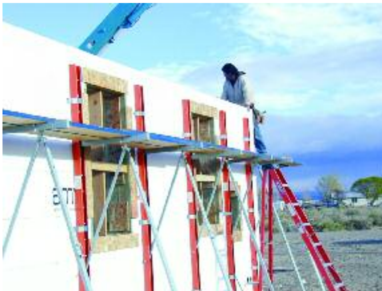
Figure 8.33 – Bracing both sides of wall openings
