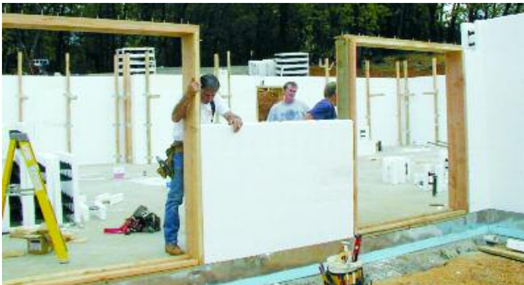
Figure 8.22 – Stacking courses around door bucks
