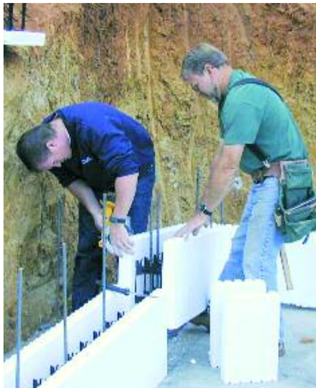
Figure 8.11 – Fitting the cut block in place
