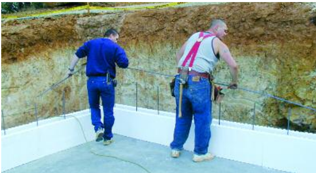
Figure 8.13 – Installing horizontal rebar
