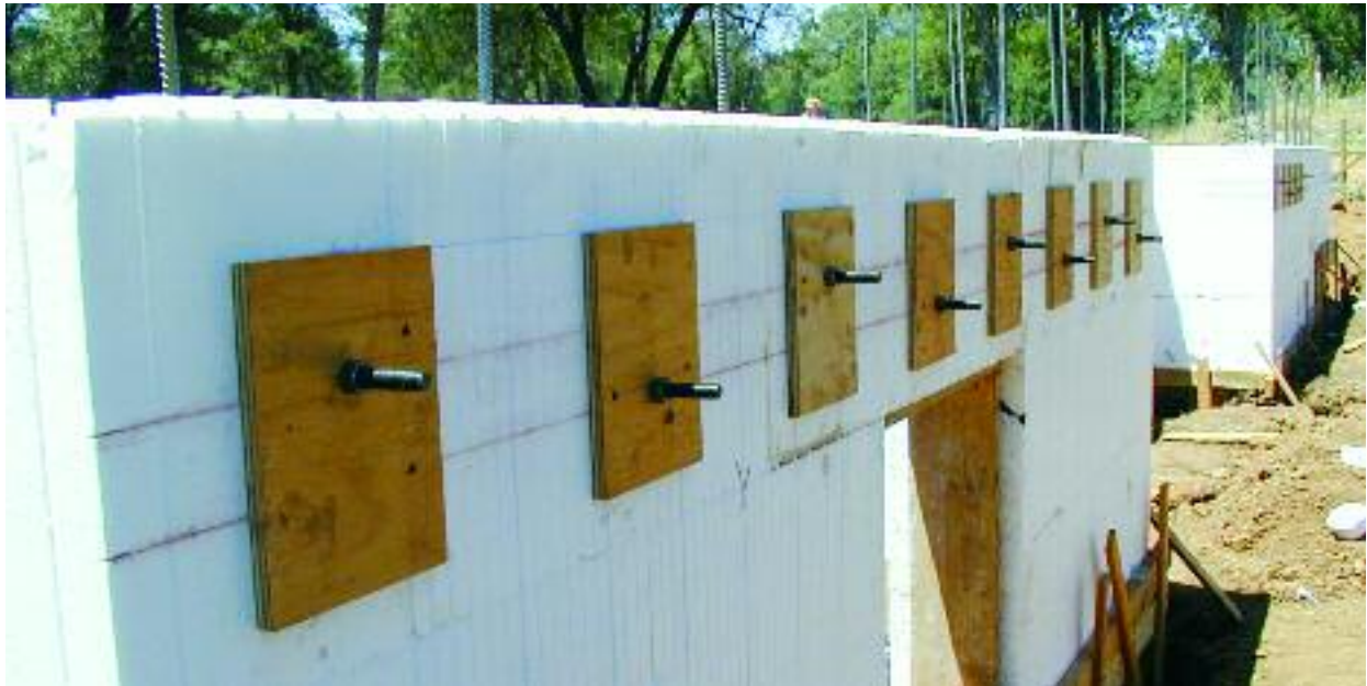
Figure 8.45 – Installing the OSB with anchor bolts onto the EPS openings and securing with sheet rock screws
