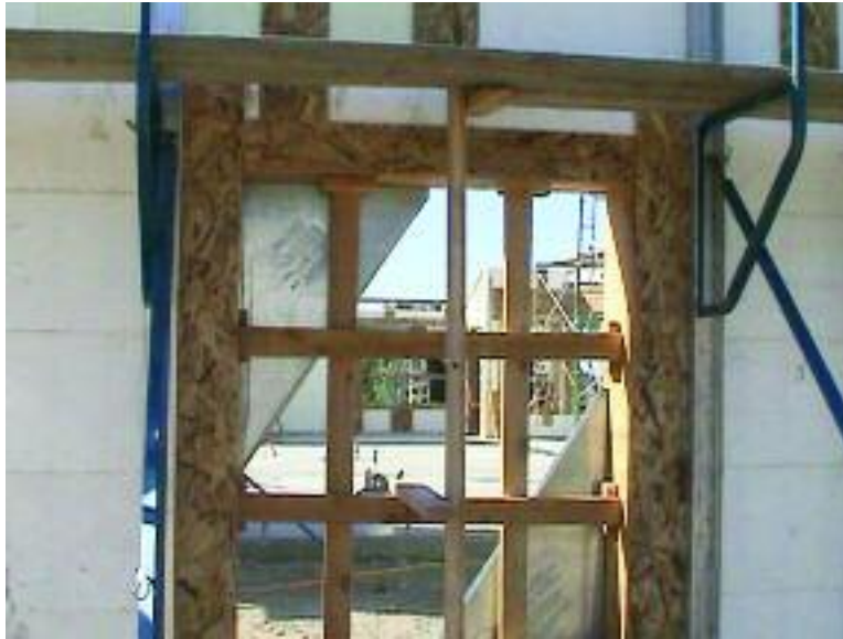
Figure 8.37 – Bracing wall opening vertically and horizontally
