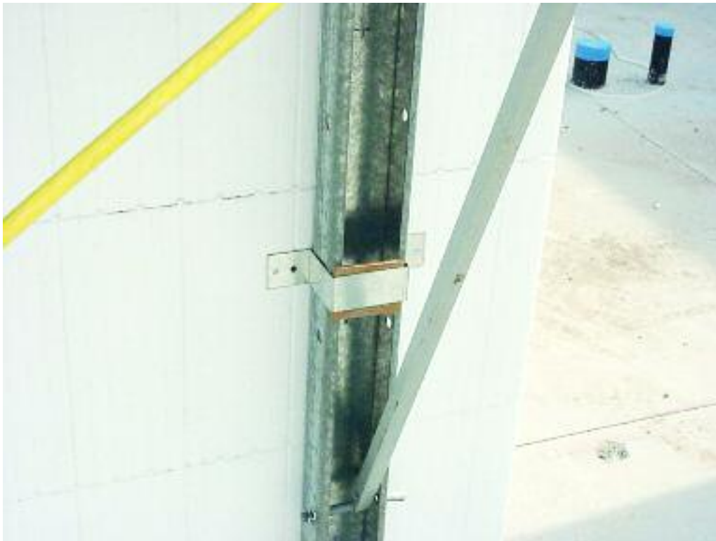
Figure 8.31 – A hat bracket wrapped around a vertical strong-back and screwed to webs on both sides
