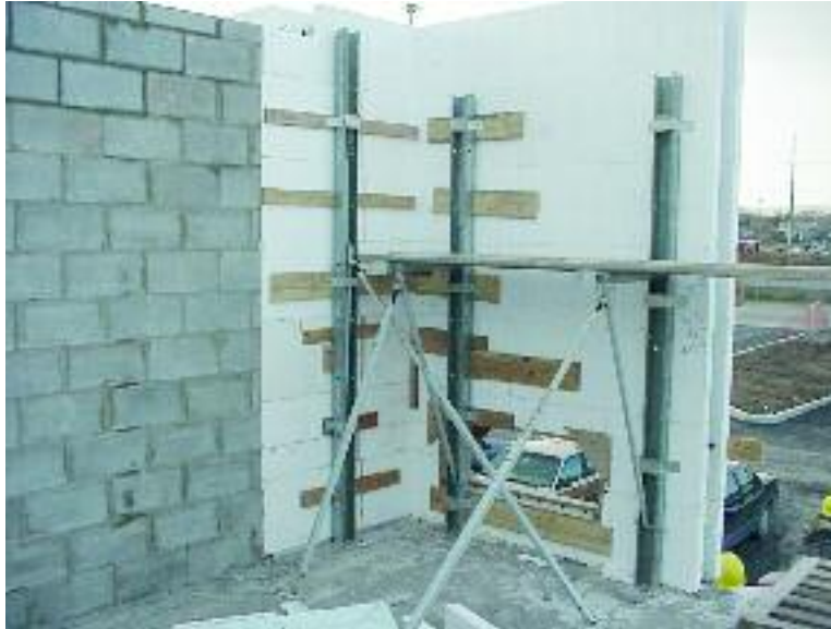
Figure 8.32 – Bracing corners on the inside
