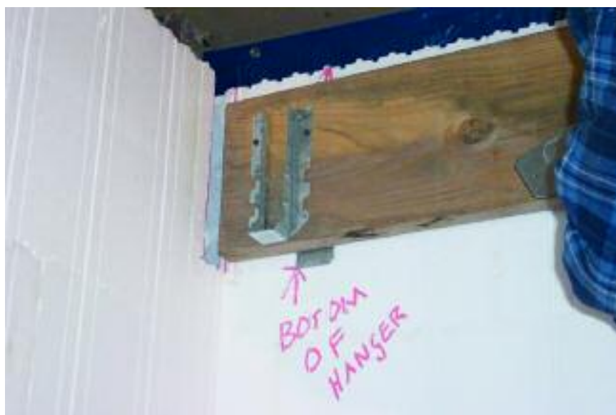
Figure 8.51 – Securing the ledger board in place temporarily
