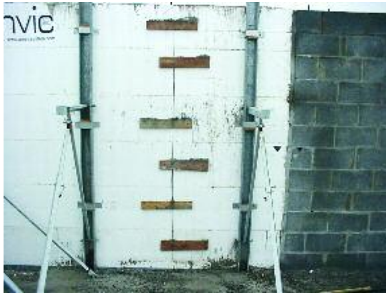
Figure 8.38 – Bracing a stack joint on both sides of wall.
