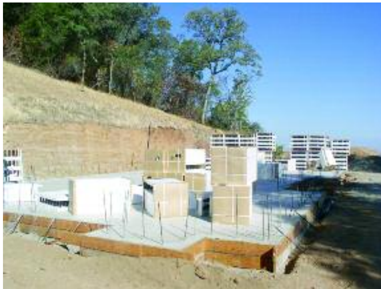
Figure 8.1 – Placing Amvic ICF within the perimeter of the wall layout
