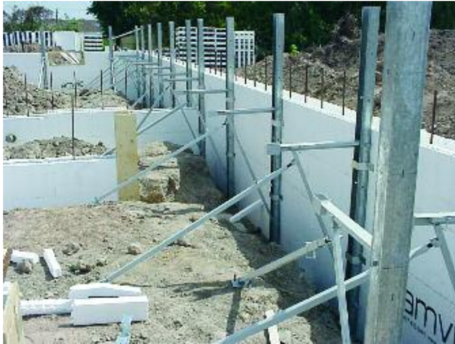
Figure 8.34 – Bracing every 6 feet
