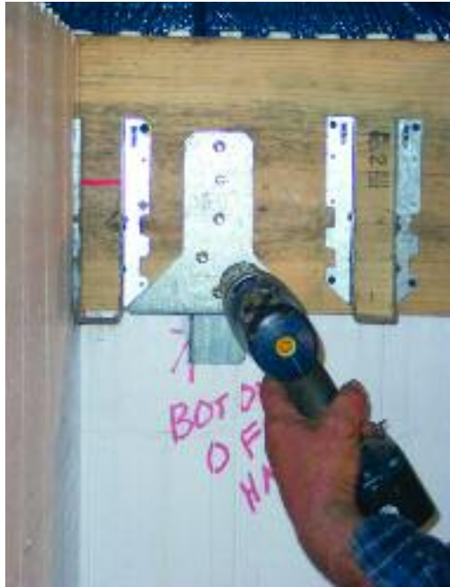
Figure 8.52 – Installing the ICFLC-W around the ledger board and drilling self tapping screws in the designated holes through to the ICFLC piece
