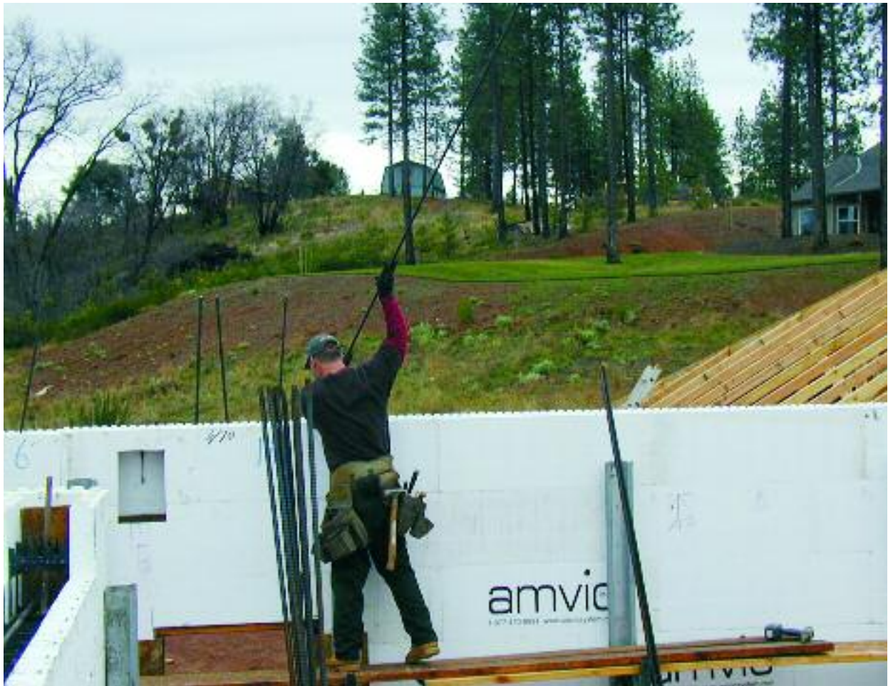
Figure 8.27 – Installing vertical reinforcing steel
