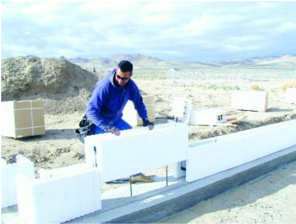
Figure 8.9 – Placing straight blocks
