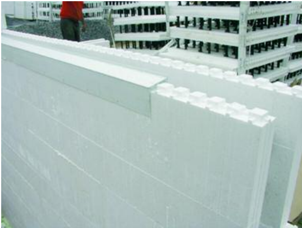
Figure 8.26 – Protecting the Interlock on a top course
