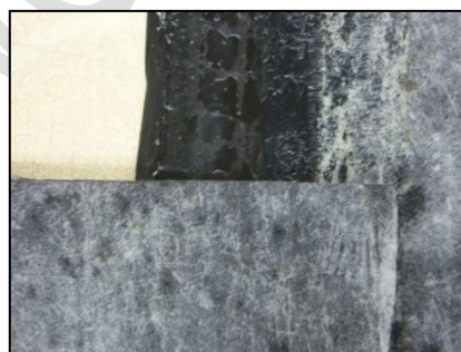
View of Overlap Seam of HydraGuard Dual Pro and HydraGuard Tile Pro
