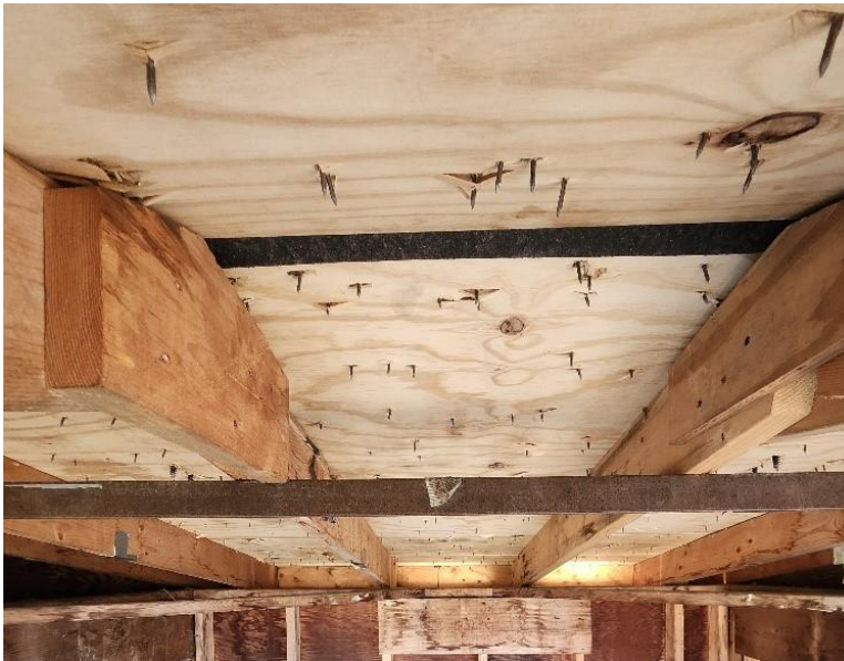
Photo No. 2 Underside Before Testing
