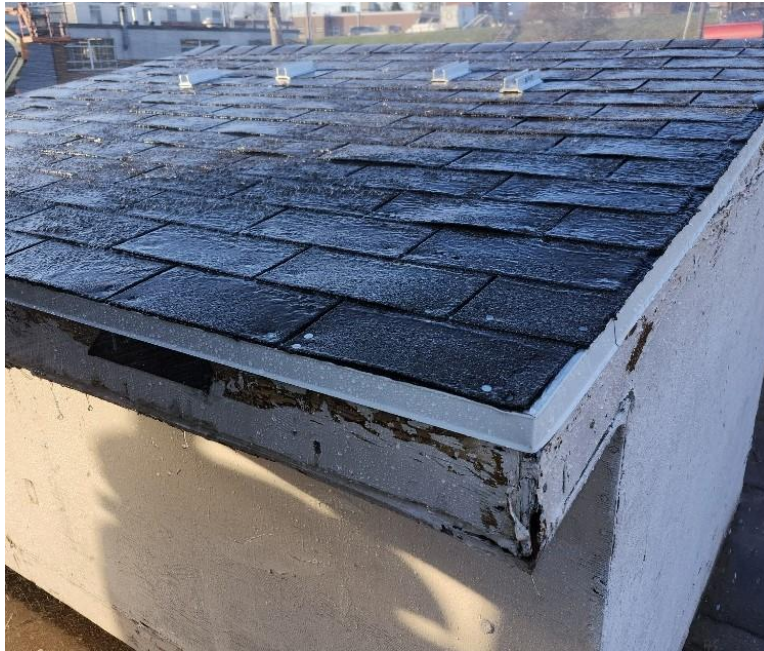
Photo No. 3 35 MPH Top Side
