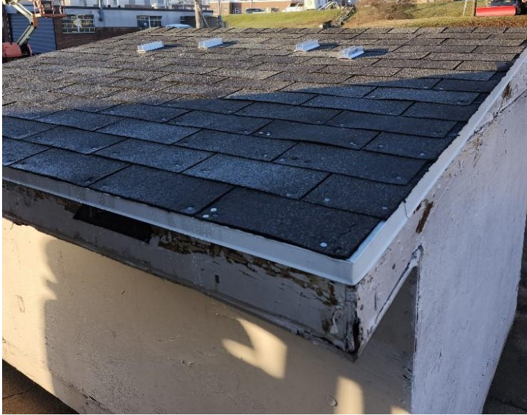
Photo No. 1 Top Side Before Testing
