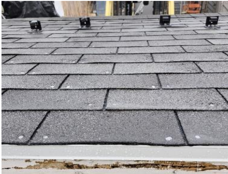
Photo No. 1 Top Side Before Testing
