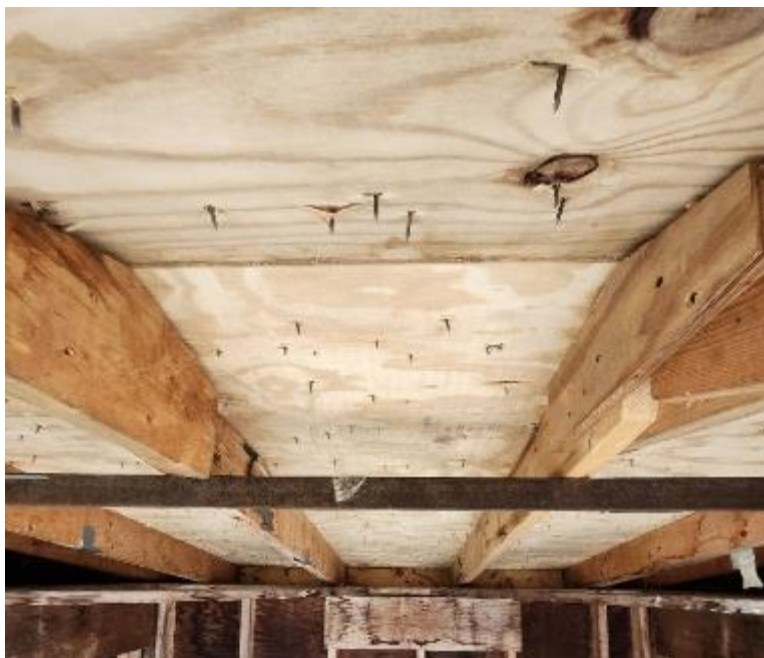
Photo No. 2 Underside Before Testing
