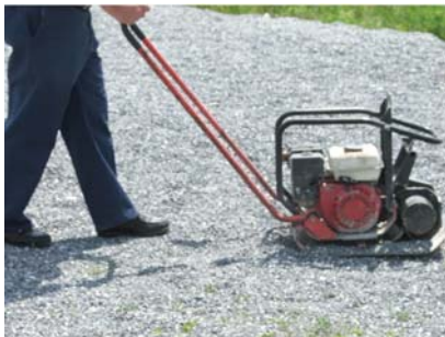
Plate Vibrator (Vibrador de Piedra) - Used to tamp stone footing prior to setting panels.
