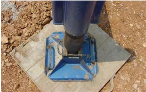
Figure 5.1 Crane outriggers must be properly blocked and supported on firm soil.
