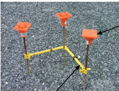
Batter Boards - Used to set up string lines which are used by Installers to properly position the panels
