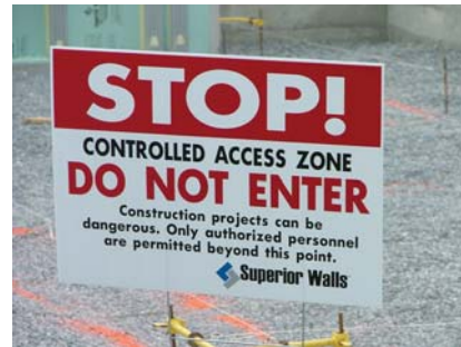
CAZ Sign (Letrero de CAZ) - Used to enforce the Controlled Access Zone at the jobsite.
