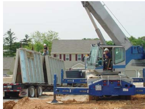
Example of a proper crane/truck pad - solid ground with no overhead obstructions.
