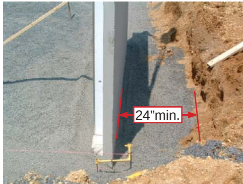
Example of a proper “over-dig”.
