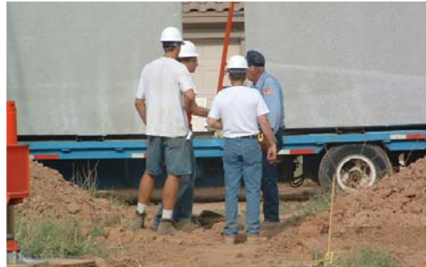
Figure 5.2 At the pre-installation huddle, crane signals, panel sequence, Controlled Access Zone and safety issues are discussed.
