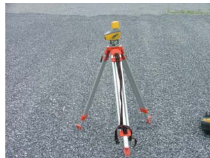
Laser Level & Tripod (Laser para Nivel) - Used to establish stone grade.
