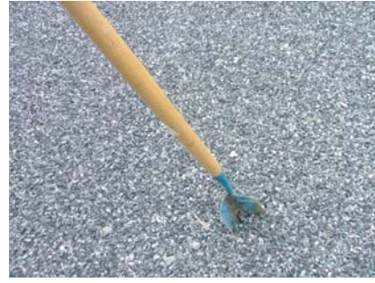
Scraper (Raspador) - Ice scraper, bent on a 45 degree angle, is used to clean loose concrete and debris from edge of panels.
