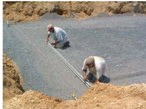
Figure 4.4 Screed stone by pulling a screed toward you. Do not use a sawing motion.
