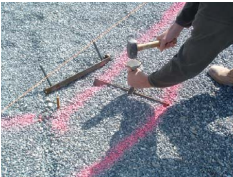
Figure 4.3 Steel angles can be used for grading blocks. Some crews prefer to use wooden blocks.
