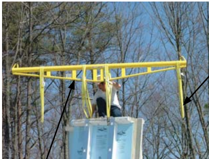
Spreader Bar (Barra de Esparciador) - Part of the lifting apparatus. Spreader Bar must be certified.
