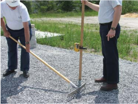
Figure 4.1 Grade stone to within 1" tolerance (of the desired finish height of stone) before tamping.
