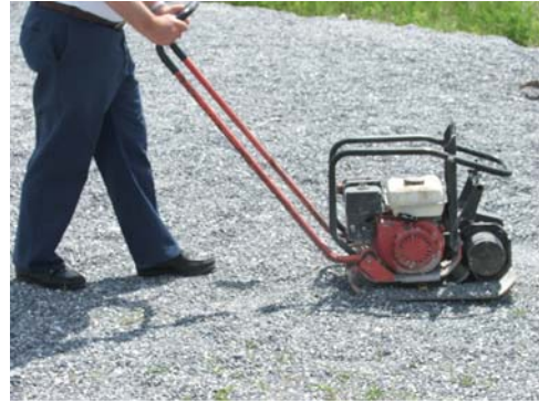
Figure 4.2 Make a minimum of three passes with a vibrating tamper.
