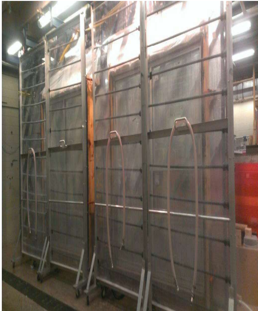
Photo No. 2 Unit During Water Infiltration
