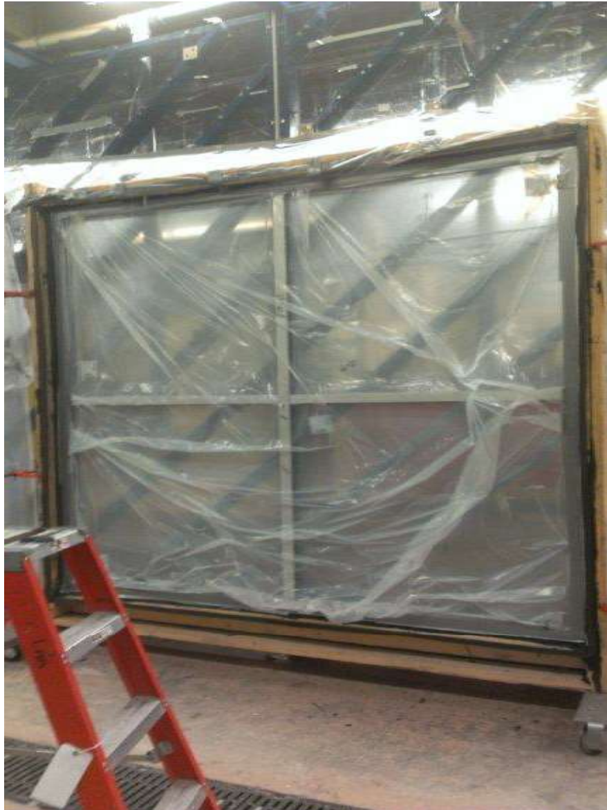
Photo No. 1 Unit During Air Infiltration
