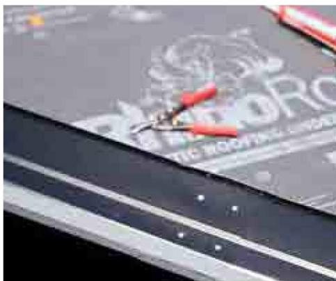
Refit the overlapping water locks together with a hand seamer.
