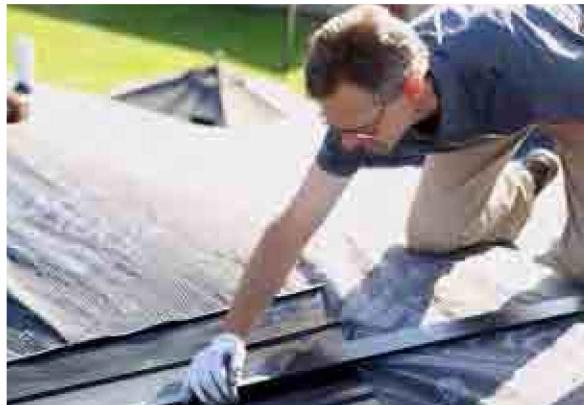
1. Install the Valley Cap by sliding it down from the top or up from the bottom. Hem to valley or secure with painted screws as necessary.
