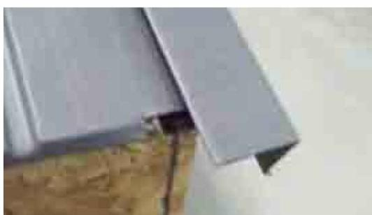
At the bottom of all trim pieces, allow for weeping of water. Panels will need to be notched out to allow water to escape.
