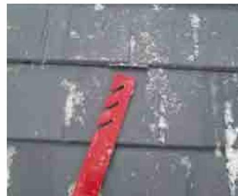
4. After panel is installed, roof jack is ready to be used. Be sure to comply with safety regulations.
