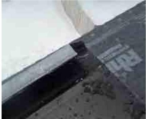
Cut bottom of inner gable so outside weeping channel will protrude past drip edge  $\frac{1}{4}$ ".
