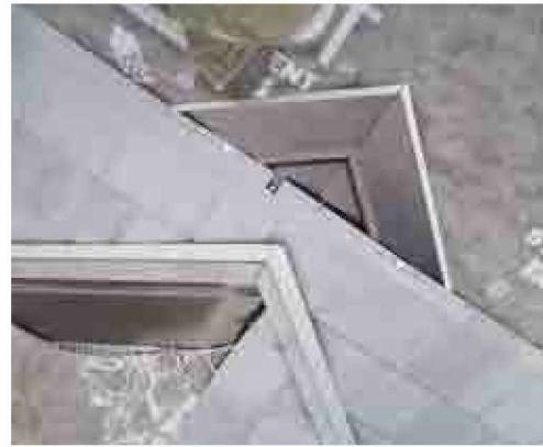
4. At the top of the valley apply sealant and install valley closure to be water tight. Apply sealant neatly and completely along all sides of the valley trim.
