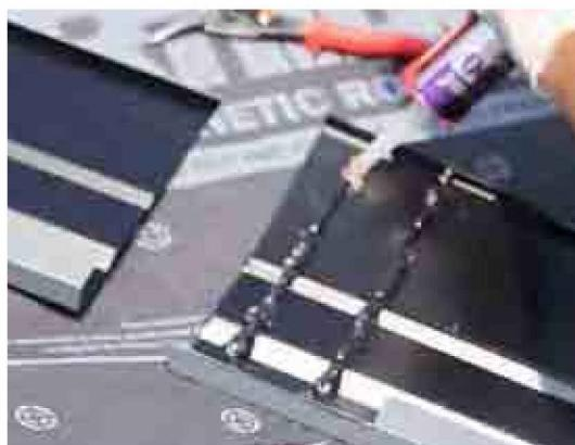
2. When overlapping, apply sealant under overlap. Be sure to screw every 12", between the diverter as shown in above diagram.
