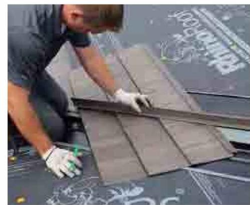
3. Cut roofing panel to match angle of Valley Closure Trim.
