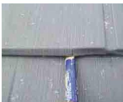
7. After sealant is applied, use a wooden tool to close and tuck flap in. Done correctly, it will be very unnoticeable from the ground.
