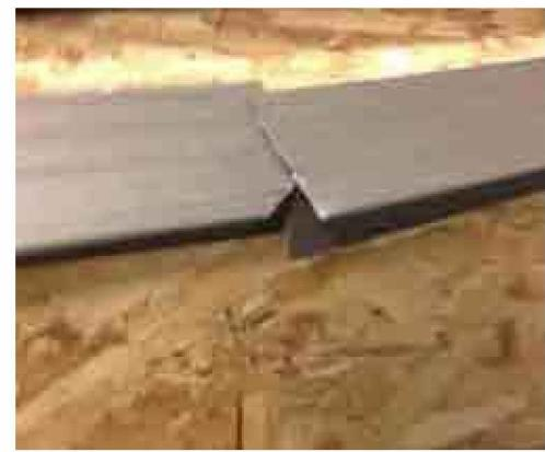
1. Cut and bend drip edge trim on the outside to conform to rake edge and inner and outer gable.
