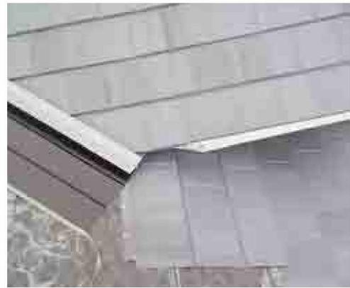
1. Install valley closure, lining up the inner diverter with the drip edge. Attach closure with screws between the two diverters.
