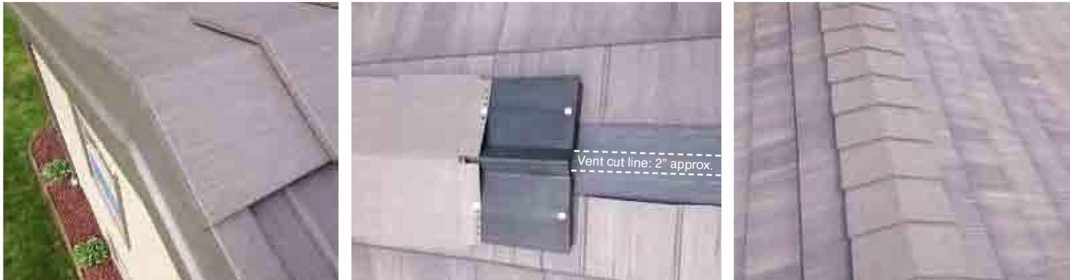
When starting ridge cap installation, bend first cap down over outer gable trim and fasten securely.
