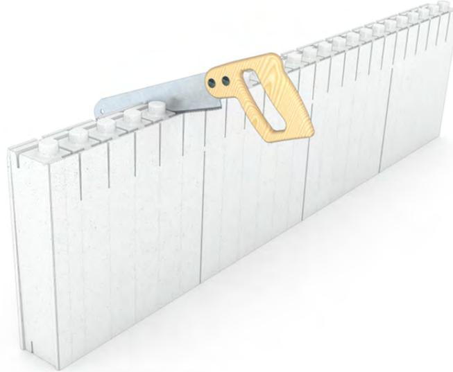
Figure 42: Cutting EPS Panels
