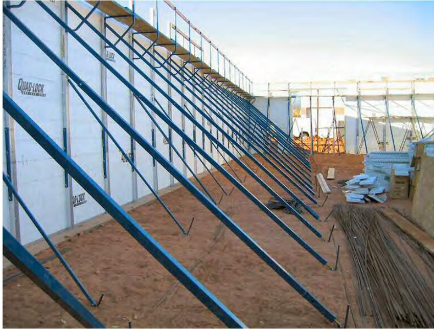
Figure 109: Bracing Tall Walls
