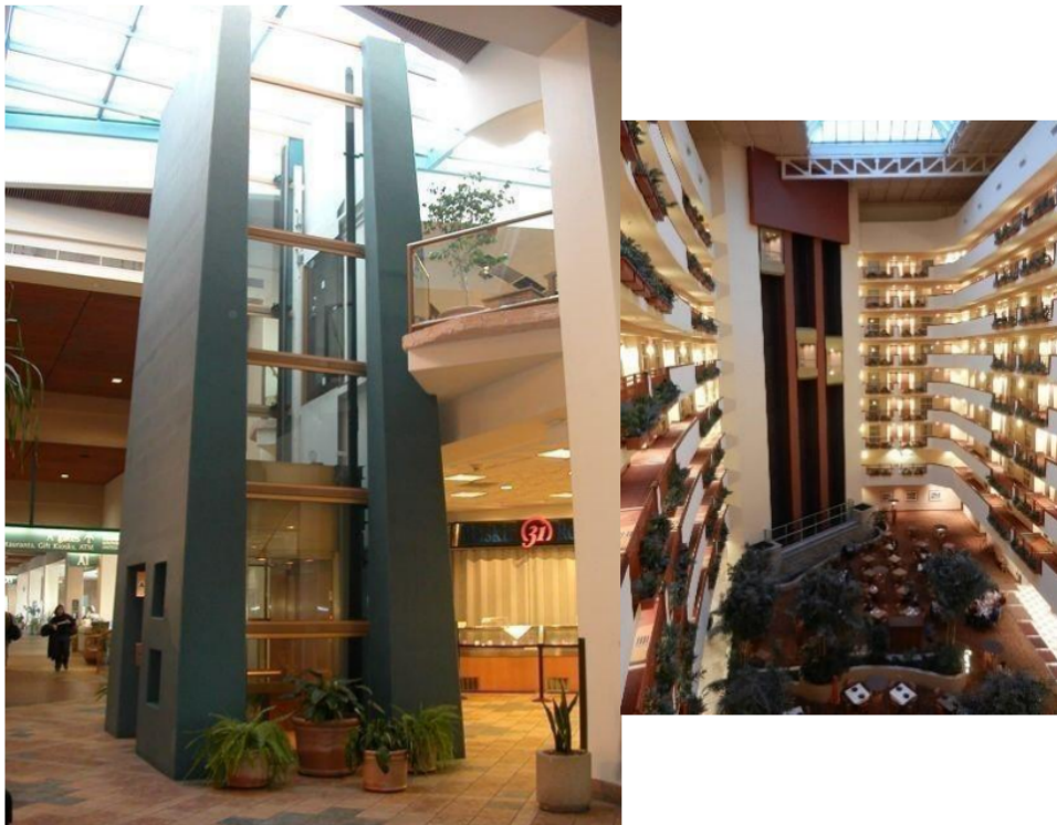
Example of elevator hoistways that are not in rated enclosures.
