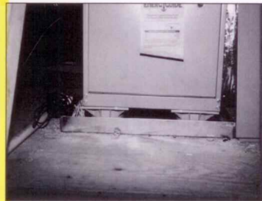
Commentary Figure 314.2.3.2 FURNACE ELEVATED ABOVE TOP OF CONDENSATE PAN
