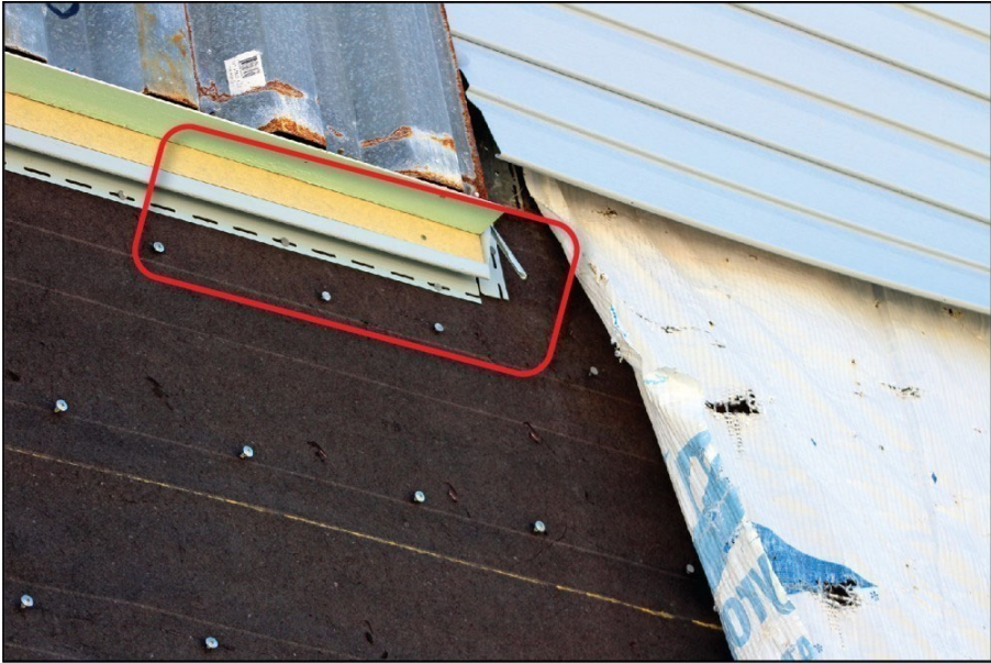
Vinyl Siding Institute (VSI) conducted several recent post-hurricane analyses and noted the need to have these requirements added to the IRC to avoid future cladding system failures. An example showing failure from Hurricane Irma that resulted from improper installation is
