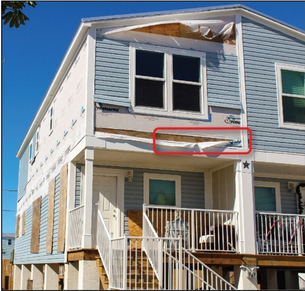
The Marathon Key house shown in the image below (FL MAT Report Figure 4-29) was permitted to have its vinyl siding replaced in 2015, with work completed in 2016. As shown in the red outline, the house appeared to lack utility trim under the window where siding was lost. Notably, the estimated maximum wind speed on Marathon Key during Hurricane Irma was 120 mph, so within the wind limitations of the IRC.
