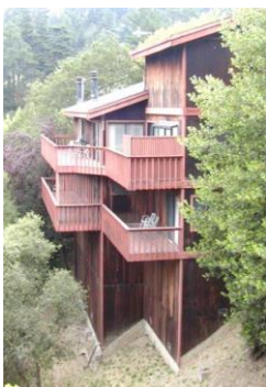
Figure 1 Hillside light-frame structure. Figure 2. Hillside structure cross-slope and out-of-hill loading.
