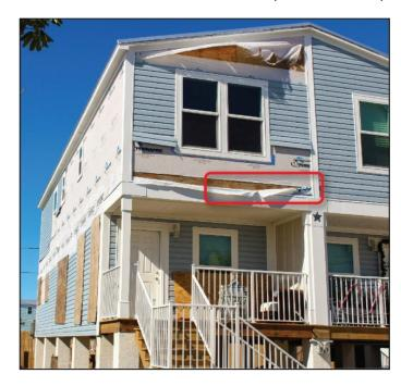
The Marathon Key house shown in the image below (FL MAT Report Figure 4-29) was permitted to have its vinyl siding replaced in 2015, completed in 2016. As shown in the red outline, the house appeared to lack utility trim under the window where the siding was lost. Notably, the estimated maximum wind speed on Marathon Key during Hurricane Irma was 120 mph, so within the wind limitations of the IRC.
