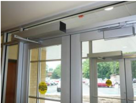
Power door operators (left doors), door closer (right door). Photo courtesy Hager Companies
