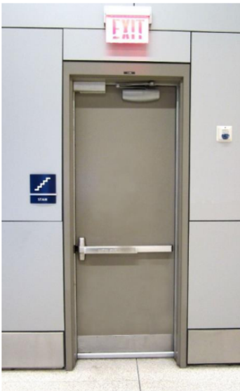
Electromagnetic door lock (top-left corner of doorway) and door closer. Photo courtesy Allegion
