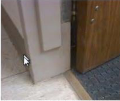
Door frame with terminated stop.
