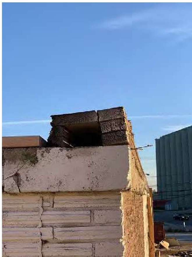
Fascia on 6" wide by 4" high "Parapet"
