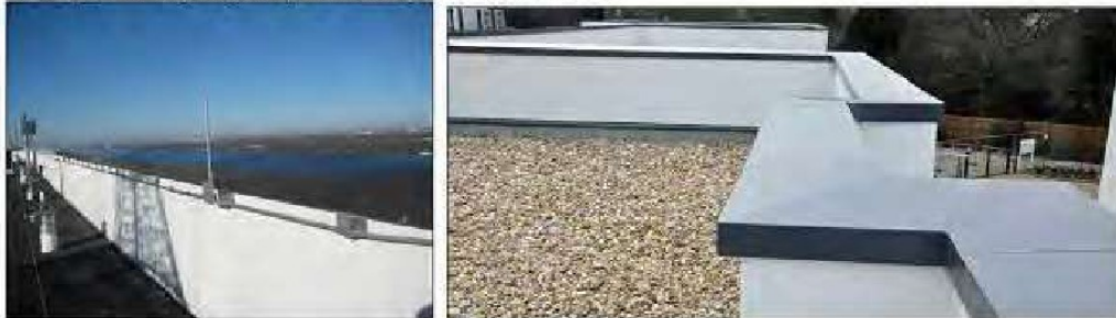
Examples of coped parapets as required by 1503.3.1.
