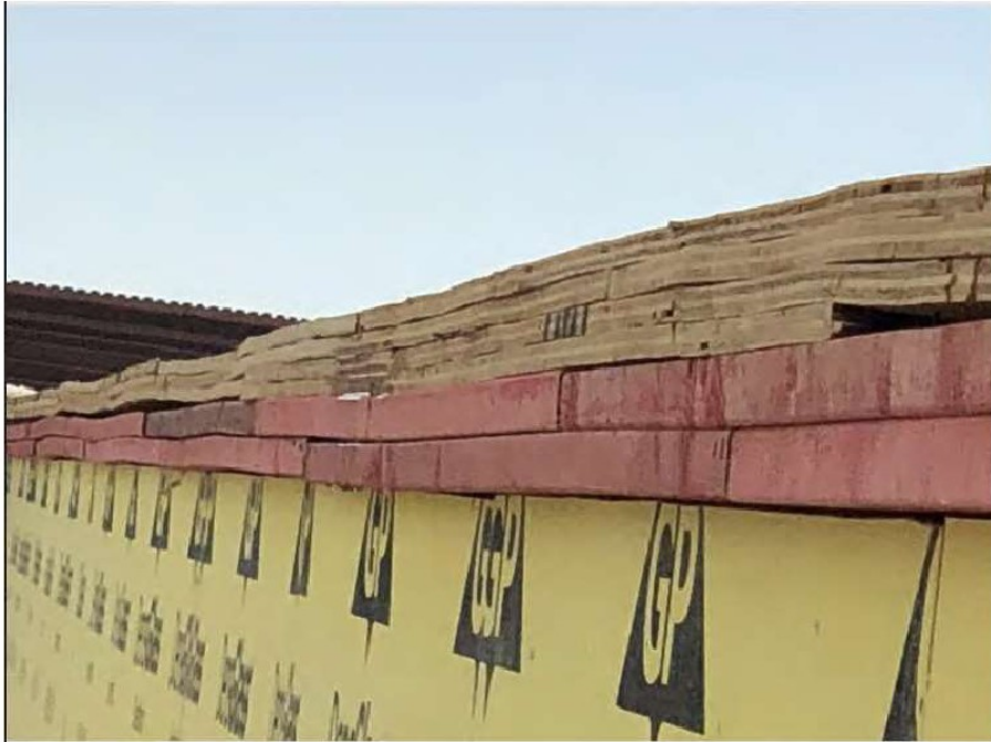
Examples of covered parapets as required by 1503.3.2.
