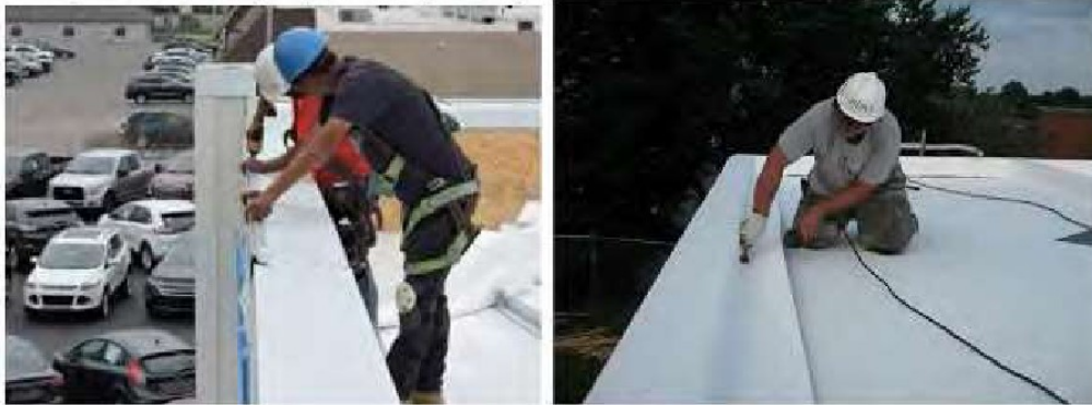
Examples of coped parapets as required by 1503.3.1.
