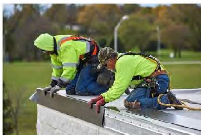
Fascia on 6" wide by 4" high "Parapet"
