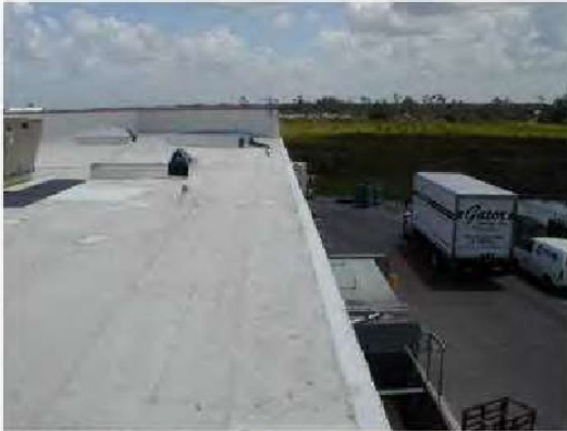
3-09-2. Large retail building. Gutter metal blew across the roof, puncturing the roof membrane and breaking skylights.
