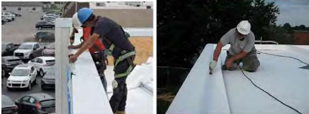
Examples of coped parapets as required by 1503.3.1.
