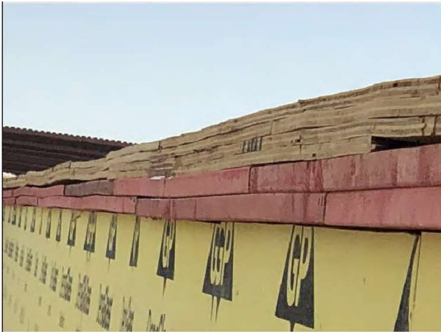
Examples of covered parapets as required by 1503.3.2.
