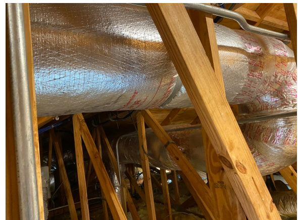
Site-wrapped supply ducts not inside the building thermal envelope must be insulated to R-8.
