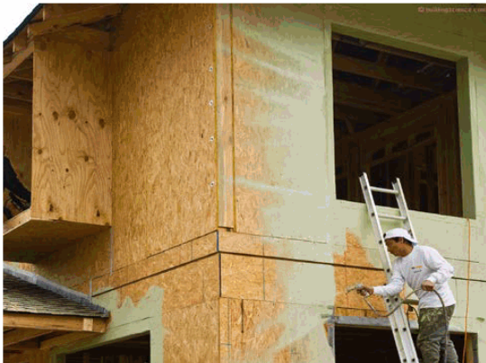
Photograph 3: Fluid Applied Membranes - Composite materials and assembly performance such as OSB covered with fluid applied water resistive barriers (WRB's) can be understood by looking at the full sorption curve. It can be argued that the wet cup properties are more significant to performance than the dry cup properties.
