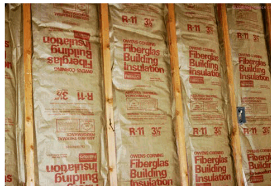
Photograph 2: Magic Valve – The asphalt coated kraft facing on the interior side of fiberglass batt cavity insulation changes its vapor transmission according to relative humidity.
