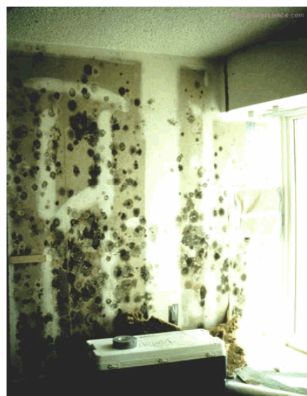
Photograph 1: Capillary Condensation and Mold - We can get condensation on porous surfaces at relative humidities less than 100 percent. The condensation occurs in the pores. Mold needs liquid phase water to do its thing yet mold happens on paper faced surfaces at 80 percent relative humidity. Thanks to Lord Kelvin and capillary condensation at 80 percent relative humidity you get liquid phase water in the pores of the paper faced gypsum due to capillary condensation.
