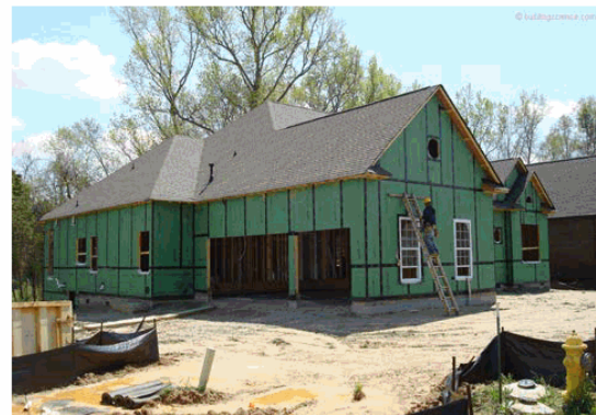
Photograph 4: Integral Water Resistive Barriers - It can be argued that the wet cup properties are more significant to performance than the dry cup properties with respect to exterior wall layers.
