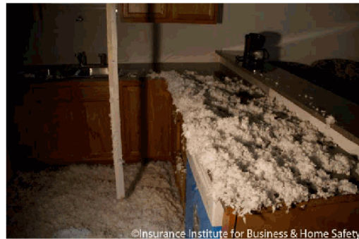
Figure 13 - Photograph of fallen portions of collapsed ceiling in the kitchen on the un-sealed roof deck side of the duplex.
