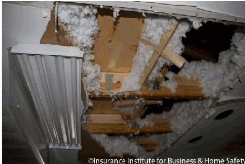
Figure 12 - Photograph of collapsed ceiling in the kitchen on the un-sealed roof deck side of the duplex.
