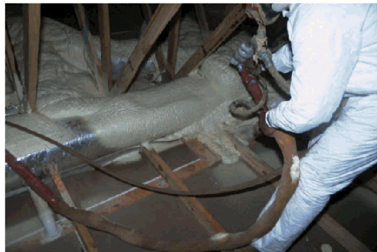
Figure 2. Ducts being encapsulated with ccSPF
