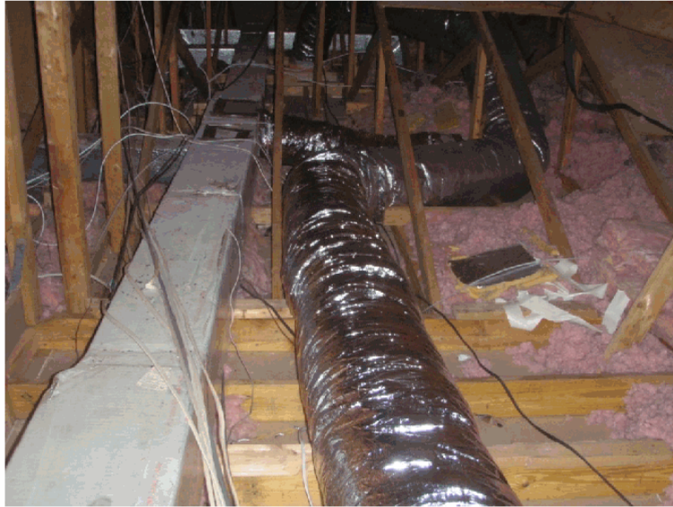
Figure 11. Duct reconfiguration at House 2
