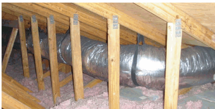
Figure 9. Return ductwork for House 2
