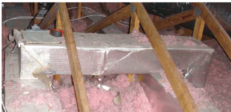
Figure 10. Supply ductwork jump over abandoned return ductwork
