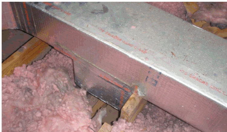
Figure 12. Open duct take-off at House 2
