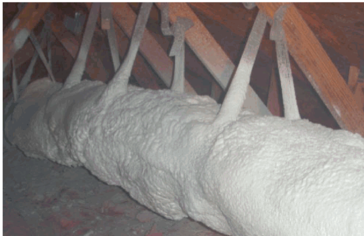
Figure 13. Finished encapsulated duct hung from roof deck
