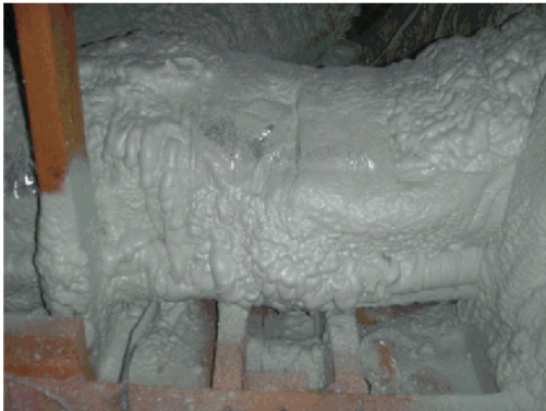
Figure 22. Varying thickness of ccSPF and interference from cross bracing
