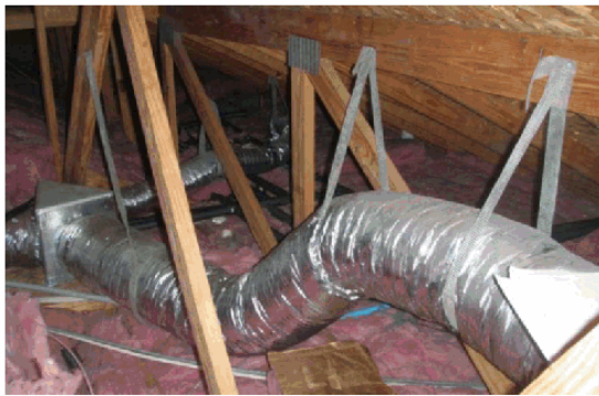
Figure 1. Traditional ductwork hung from attic rafters
