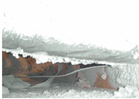
Figure 19. Exposed underside of ductwork not adequately covered with ccSPF
