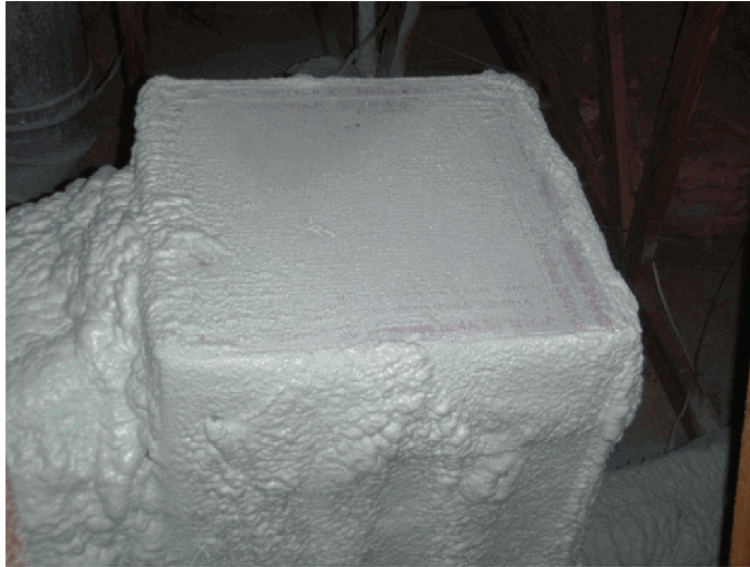
Figure 17. Improperly spray-foamed plenum box at House 1
