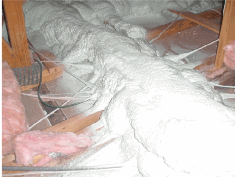
Figure 16. Electrical, telephone, and other wiring permanently spray foamed to the ceiling and ductwork during retrofit
