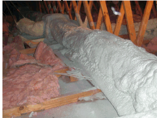
Figure 21. Rigid insulation inserted under ductwork to serve as a substrate and provide insulating value
