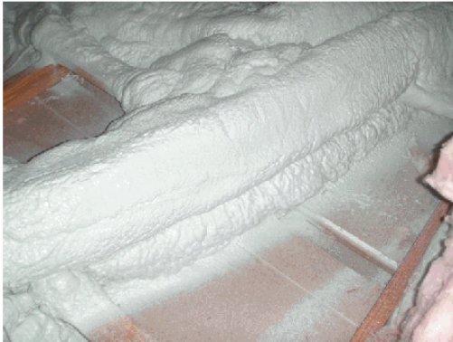
Figure 20. Ductwork well-sealed to sheetrock with ccSPF
