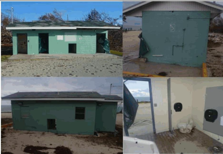
Figure 5. Florida, after Hurricane Irma, flood Zone V. No evidence of structural damage after estimated 5 ft stillwater plus waves. From upper left: facing beach, side, interior, rear.
