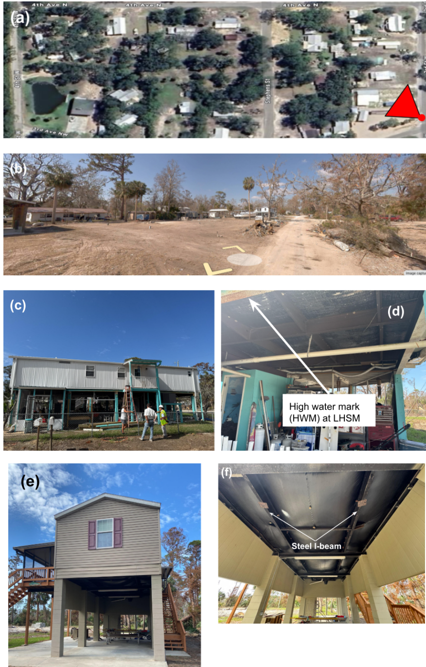
Figure 18. Performance of RVs and manufactured homes during Hurricane Helene in Steinhatchee, FL: (a) pre-storm and (b) post-storm views of a manufactured home park; The red triangle in (a) approximates the location of streetview in (b); (c) an elevated manufactured home built in 2001 with an 8-ft elevation to the LHSM survived, while neighboring slab-on-grade homes were washed away; (d) high water mark (HWM) reaching the LHSM, preserving the contents of the livable floor in the same home; (e) another elevated manufactured home, built in 2004 with an 11-ft elevation to the LHSM; and (f) the higher freeboard in this home prevented surge and wave exposure to the steel I-beam LHSM.
