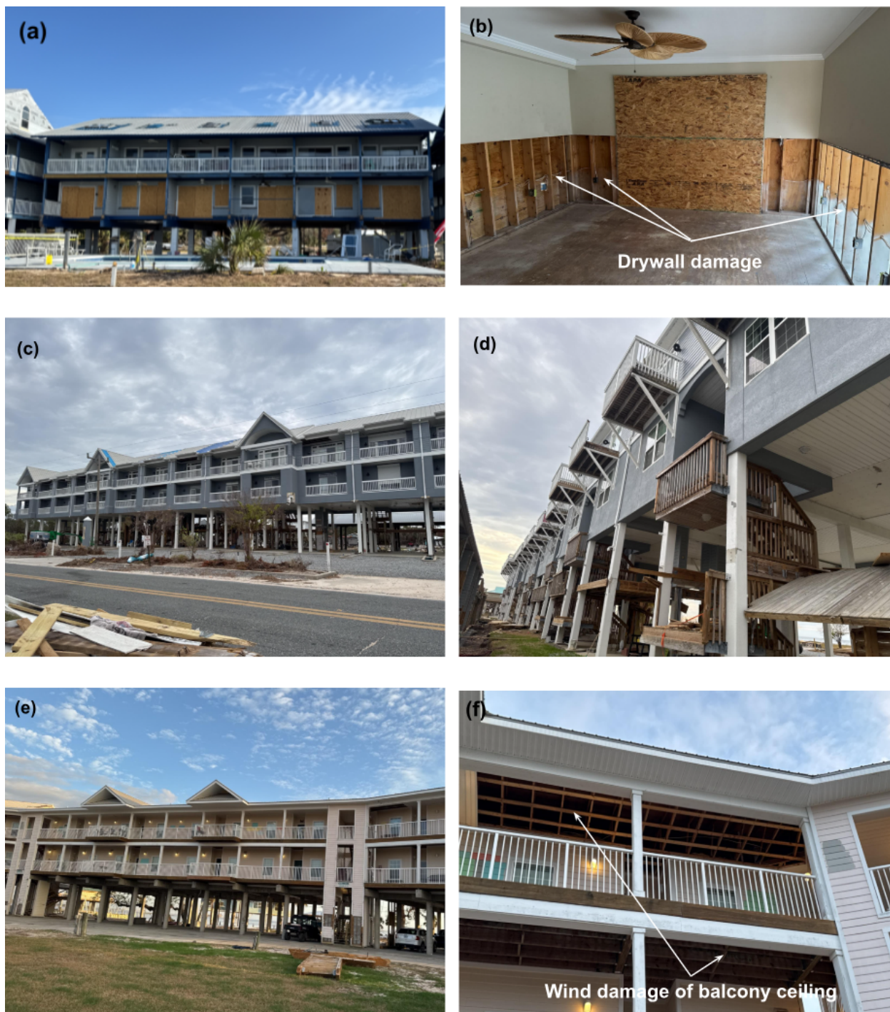
Figure 15. Performance of multi-family condos during Hurricane Helene: (a) substantial to heavy damage to a condo built in 2007 near the Steinhatchee Marina, elevated on an 8-foot wooden foundation and (b) interior view of a second-story room showing water damage to the drywall of that condo; (c) minimal structural damage to a condo on Keaton Beach Rd, built in 2005 on 18-foot concrete columns to the lowest horizontal structural member (LHSM); however, wave and surge damage primarily affected the (d) ground-floor utility enclosure and stairway decks; (e) a multi-family condo on Main Street in Horseshoe Beach, built in 2005 on 12-foot concrete piers
