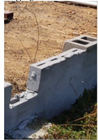
Unreinforced masonry stem wall
