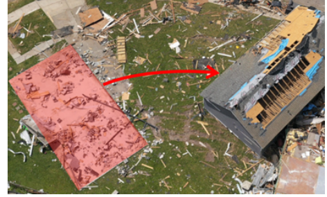
(c) Shifted off foundation
