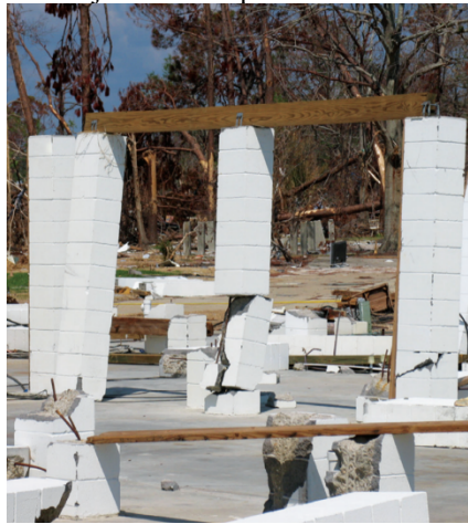
Reinforced masonry piers. Note the presence of rebar in the columns.
