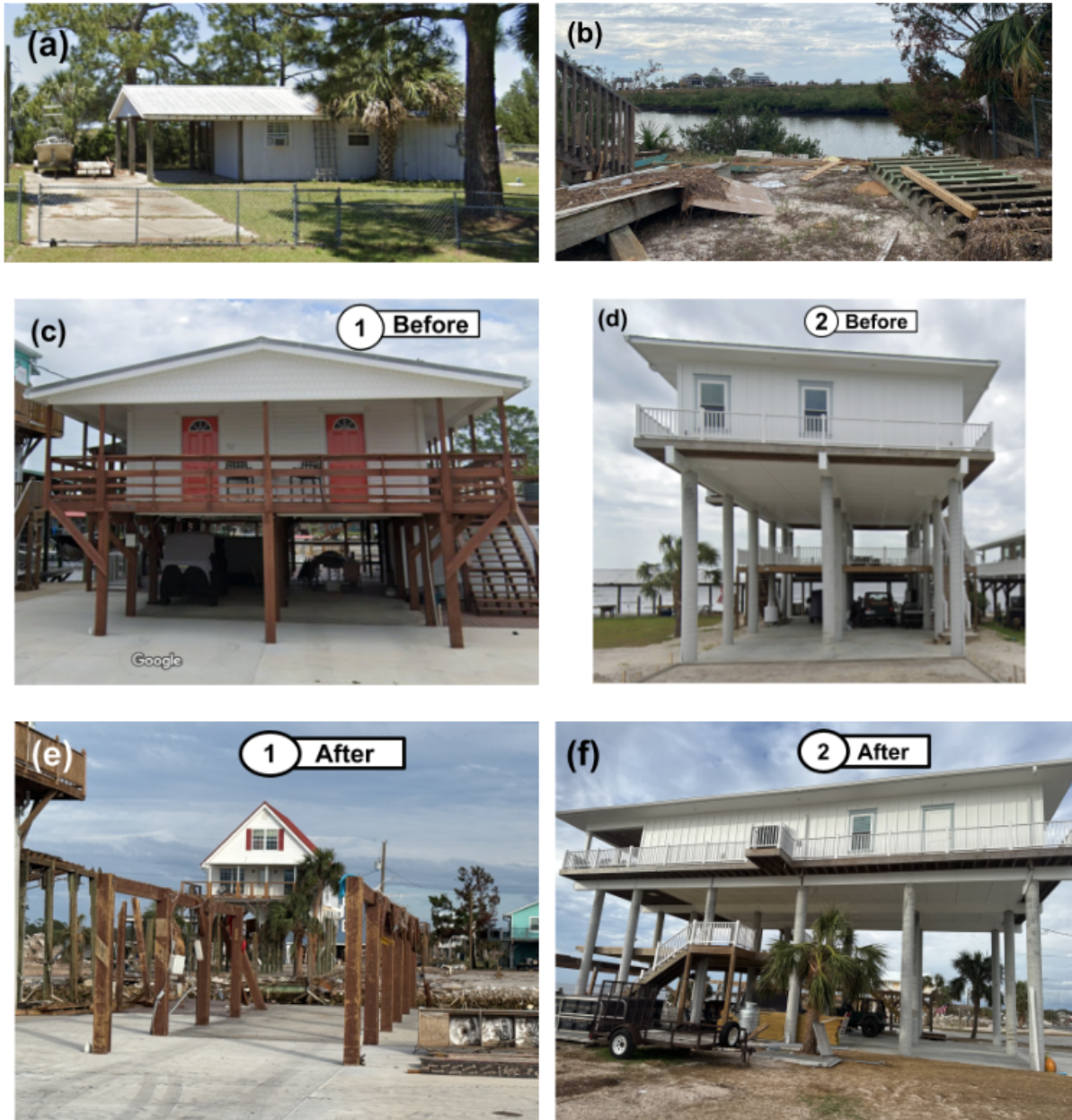
Figure 14. Impact of floor elevation on the survivability of coastal homes: (a) pre-storm and (b) post-storm views of a slab-on-grade single-family home on Dekle Beach Blvd, built in 1996, which was completely washed away during Hurricane Helene; (c, d) pre-storm and (e, f) post-storm views showing the contrasting performance of two elevated homes on Keaton Beach Rd, FL. Home (1), built in 2000, features wooden columns with a 7-foot elevation to the lowest horizontal structural member (LHSM), whereas home (2), constructed in 1977, is supported by cast-in-place concrete columns with a 20-foot elevation to the LHSM.
