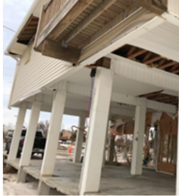
Cast-in-place concrete piers. No joints in the piers are visible.
