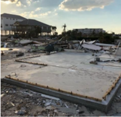
Concrete slab-on grade
