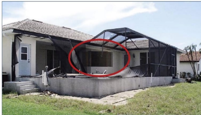
Figure 14. Broken window from debris (in the red circle) caused by Hurricane Charley (2004), in Punta Gorda.
