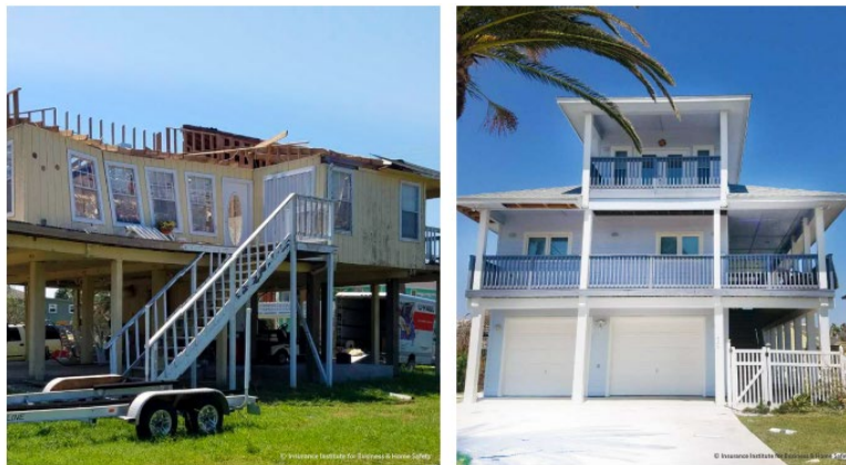
Figure 35. Port Aransas North: Two homes located 250 ft apart that experienced similar wind speeds during hurricane Harvey (2017). 1987 construction (left), 2006 construction (right).
