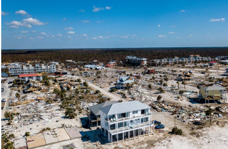
Figure 45. Widespread devastation to wood-framed single and multi-family residences in Mexico Beach with few survivors in areas with highest inundations (Source: New York Times)
