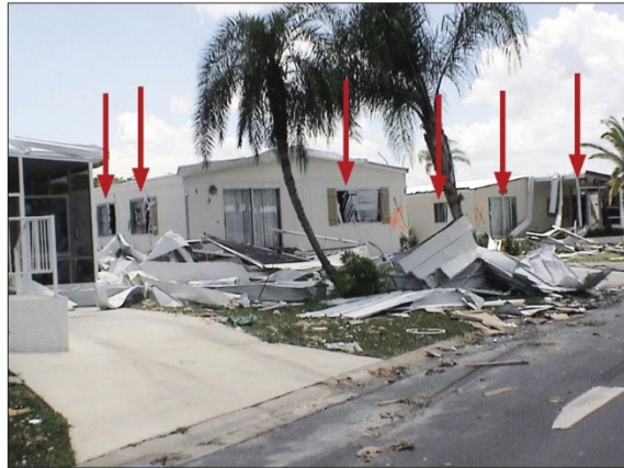
Figure 11. Wind-borne debris damage on windows caused metal roof panel and siding in Port Charlotte during Hurricane Charley (2004).
