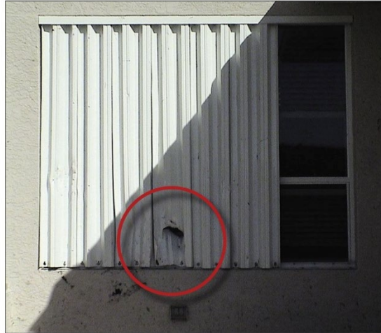
Figure 6. A roof tile punctured a Miami-Dade County approved shutter in Punta Gorda Florida during Hurricane Charley (2004).
