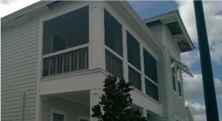
Figure A-12: 13 Smiling Fish Lane Damaged Soffits (Site 2)
