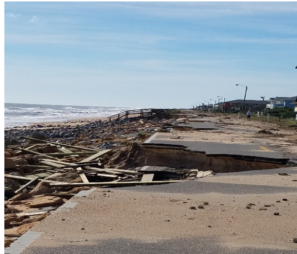
Figure A-2: Damage to A1A in Flagler Beach, FL
