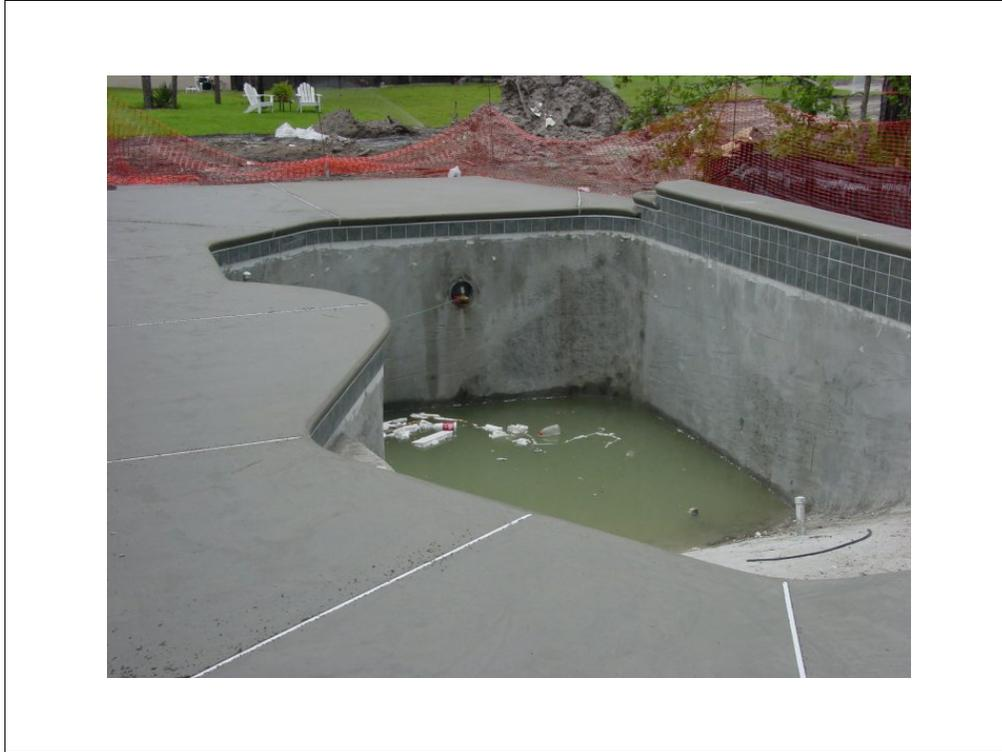
Freshly poured pool deck showing expansion joints.
