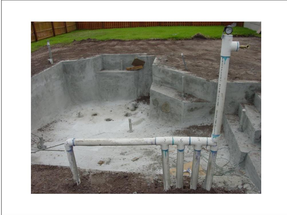
Pressure test on manifold for infloor cleaning system.
