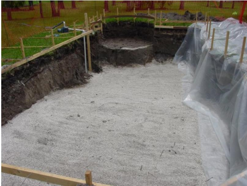
Notice visqueen protecting “wall” of pool from rain events. Also, chat rock placed in bottom (not required).
