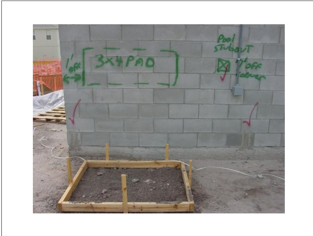
Check to see there is no service panel behind electrical stub out for pool. Also, that there is a clear area for working on the equipment.
