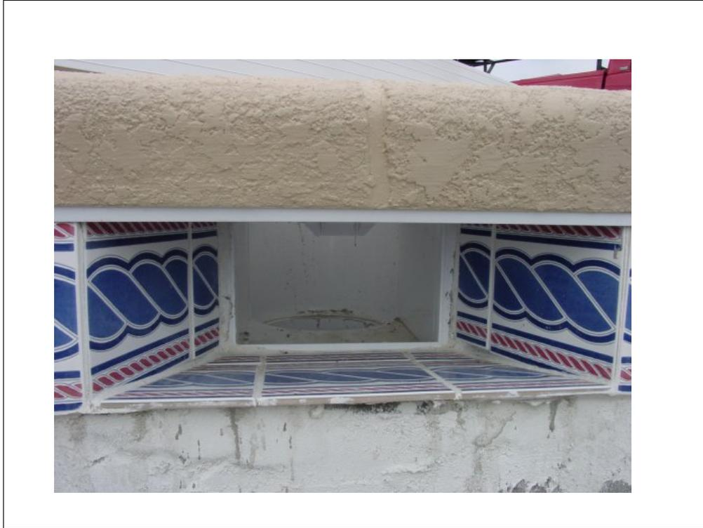
Check skimmer. Distance to skimmer from back of beam depends on manufacturer. In this case, the distance to the water's edge from front of skimmer is 8" with a 9" opening and an approximate 20" flange.
