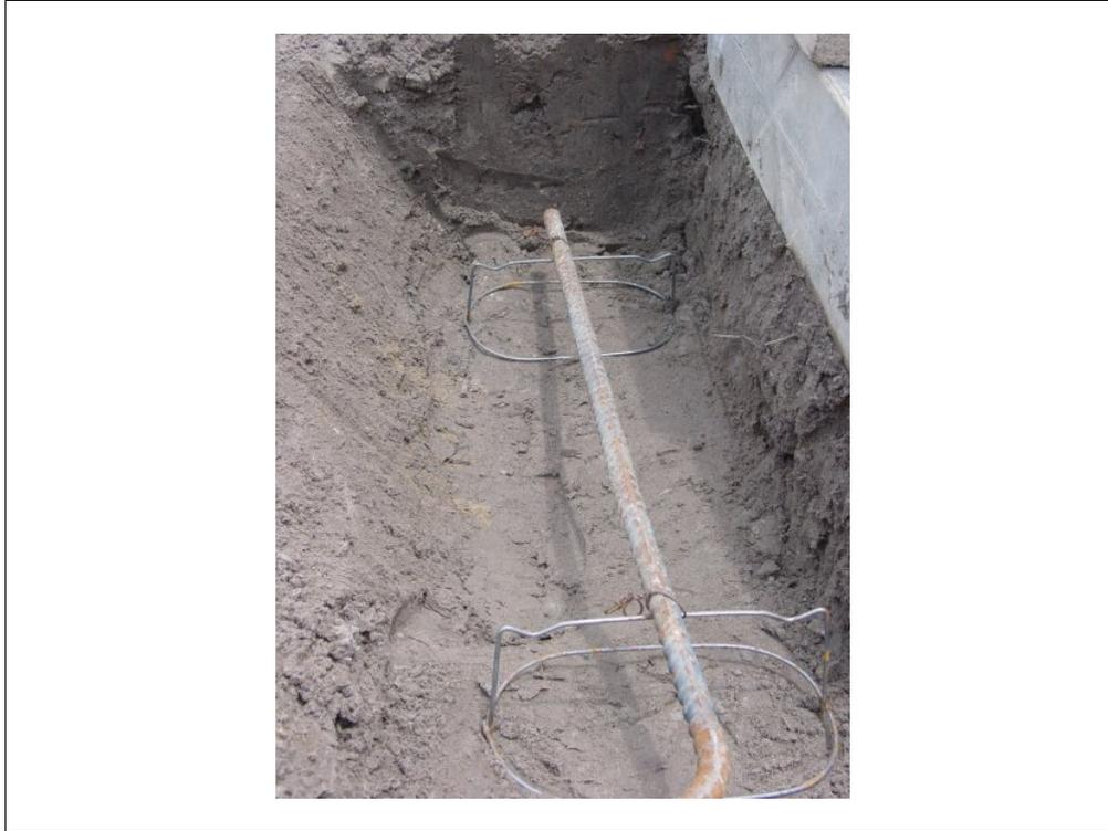
Check footing for screen enclosure, which is dependent on size of screen enclosure. In this instance, #5 (5/8") rebar was required.
