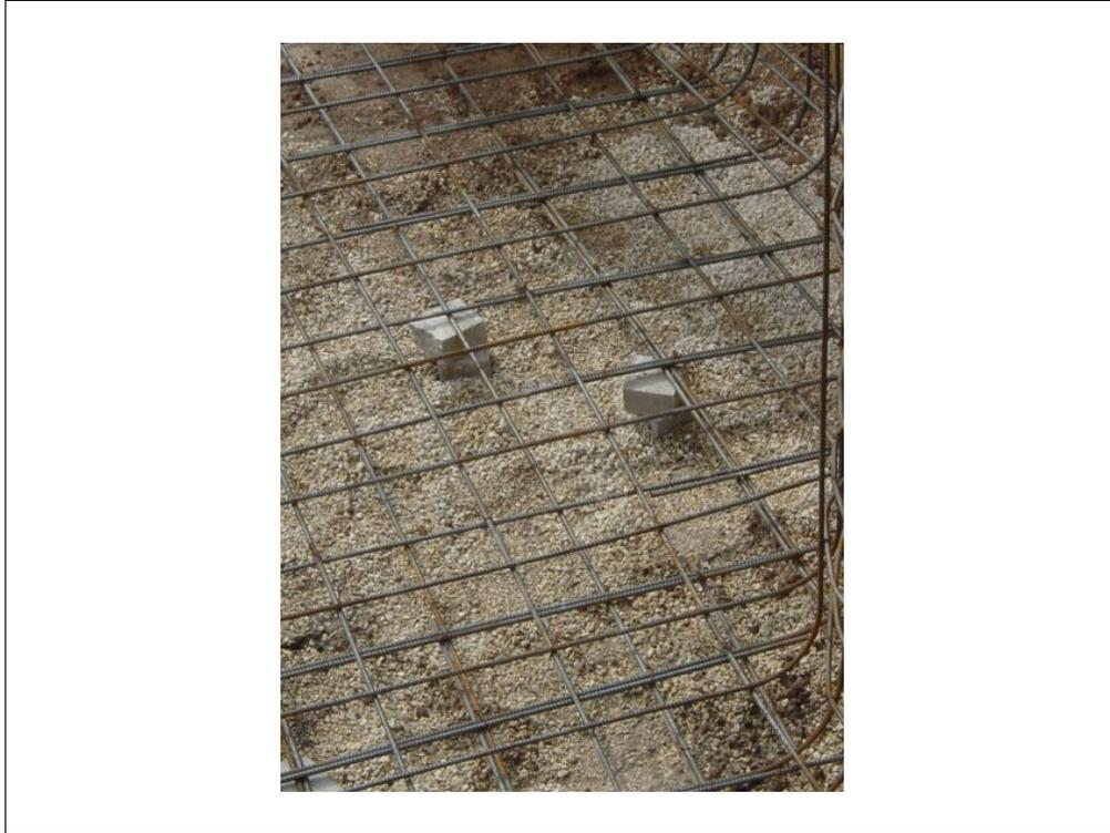
This image depicts lap on rebar, ties, and steel elevation.
