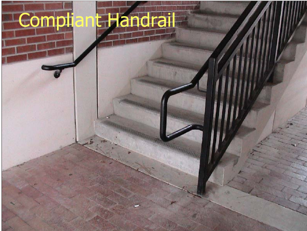
Stairs with compliant handrails
