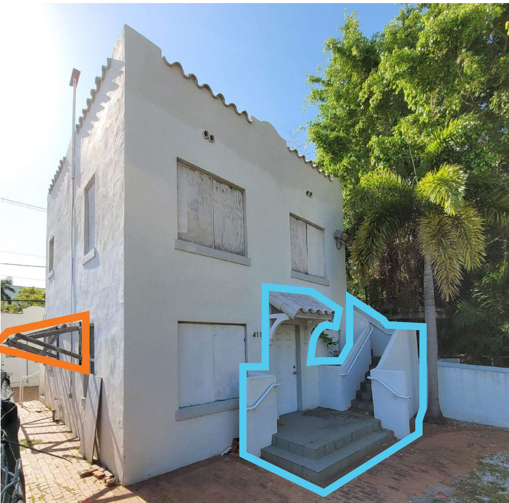
WOOD TRELLIS - TO BE REMOVED FRONT ENTRY & STAIR - TO BE REPLACED
