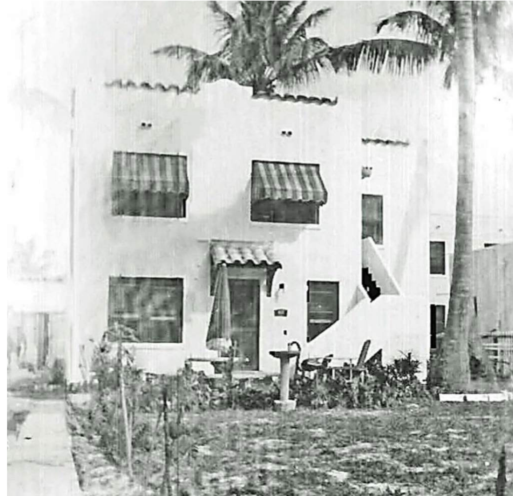
ORIGINAL HISTORIC BUILDING, 1955
