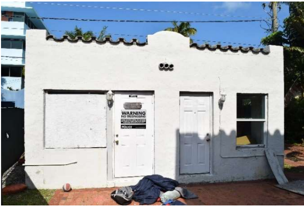
Fig. 25. Front façade of secondary building, May 2021.
