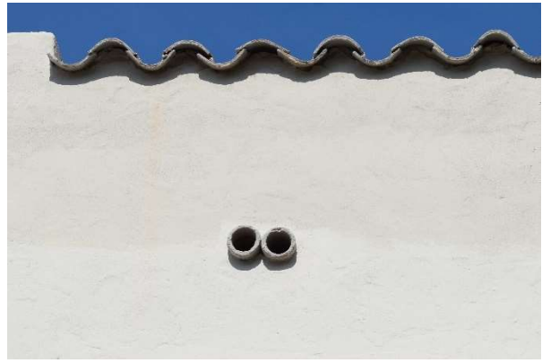
Fig. 17. Detail of paired attic vent tubes at front façade, May 2021.
