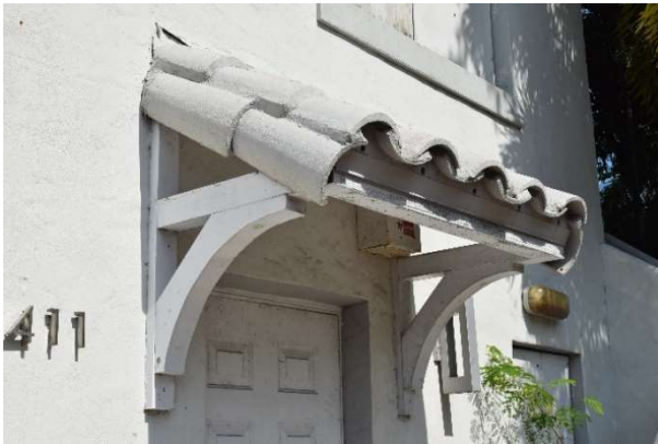
Fig. 18. Detail of pent roof with barrel tile and knee braces at entrance door, May 2021.
