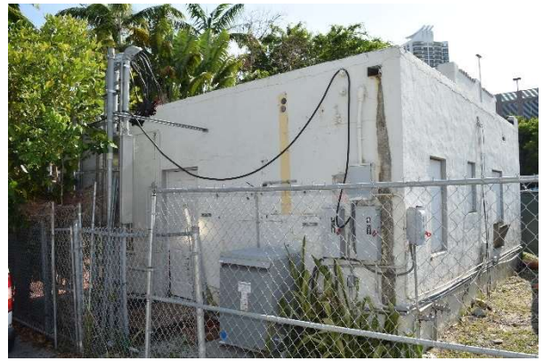
Fig. 26. North and east elevations of secondary building, May 2021.
