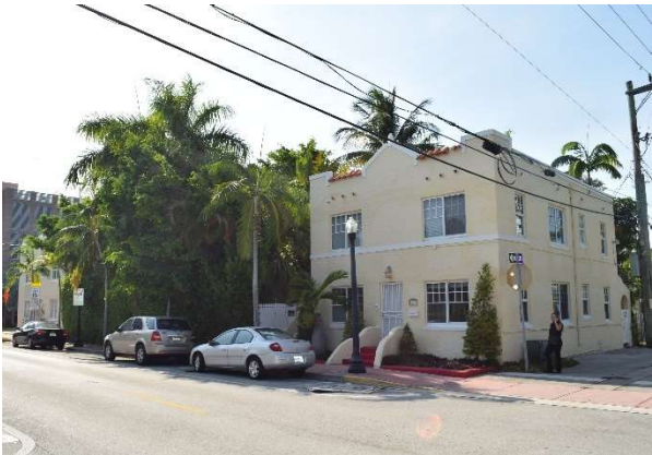
Fig. 10. Buildings facing 4 th Street, south of the site, May 2021.
