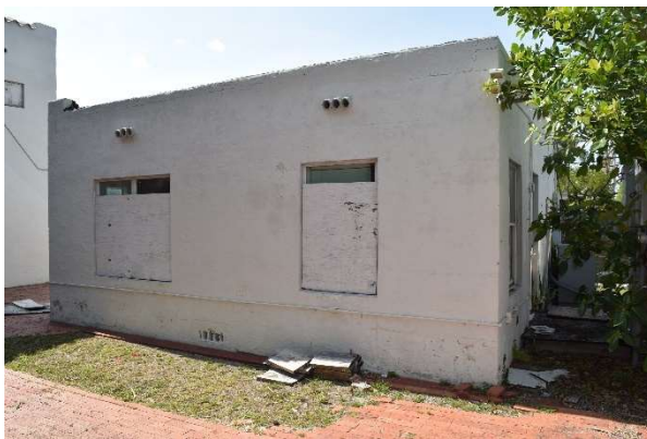
Fig. 27. South elevation of secondary building, May 2021.
