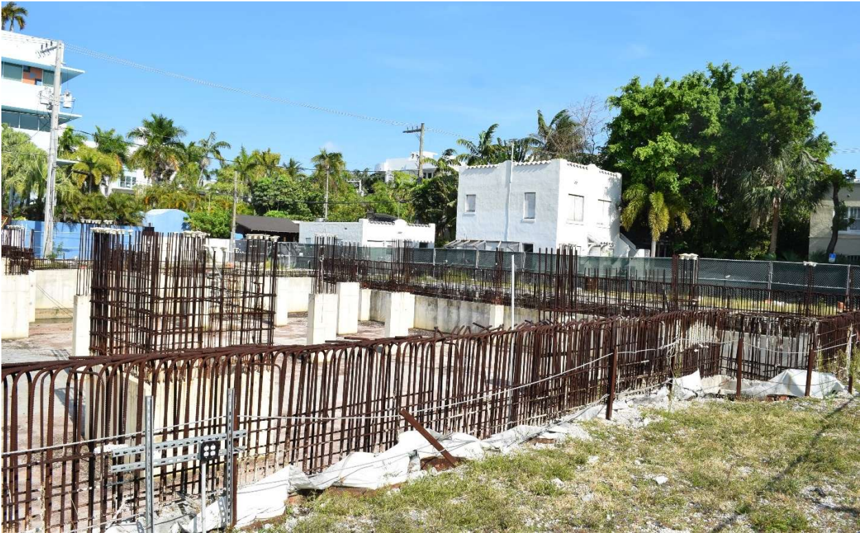
Fig. 9. Abandoned construction site immediately north of 411 Michigan Avenue, May 2021.
