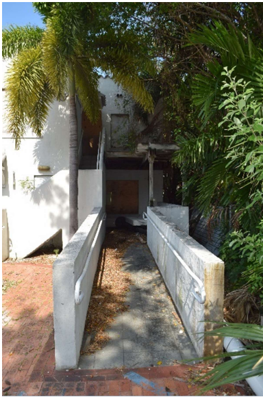
Fig. 20. Detail of accessible ramp, May 2021.
