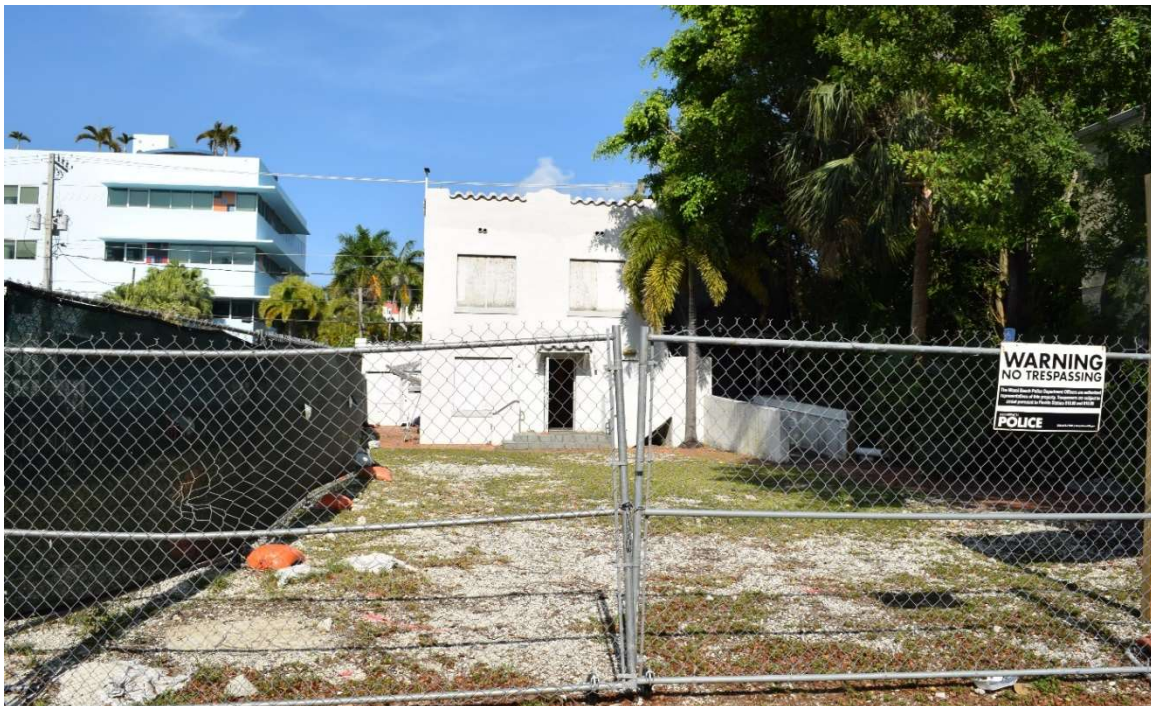
Fig. 14. View of the site looking east from Michigan Avenue, May 2021.
