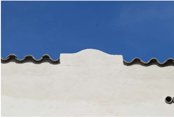
Fig. 16. Detail of scalloped parapet at front façade, May 2021.
