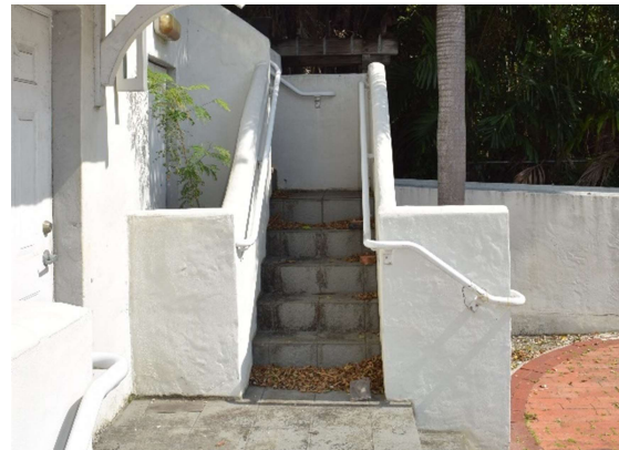
Fig. 19. Detail of stair to 2nd Level, May 2021.
