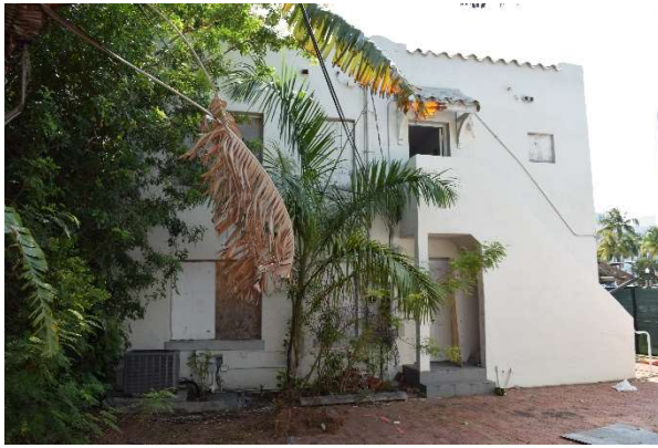
Fig. 23. View of east elevation, May 2021.
