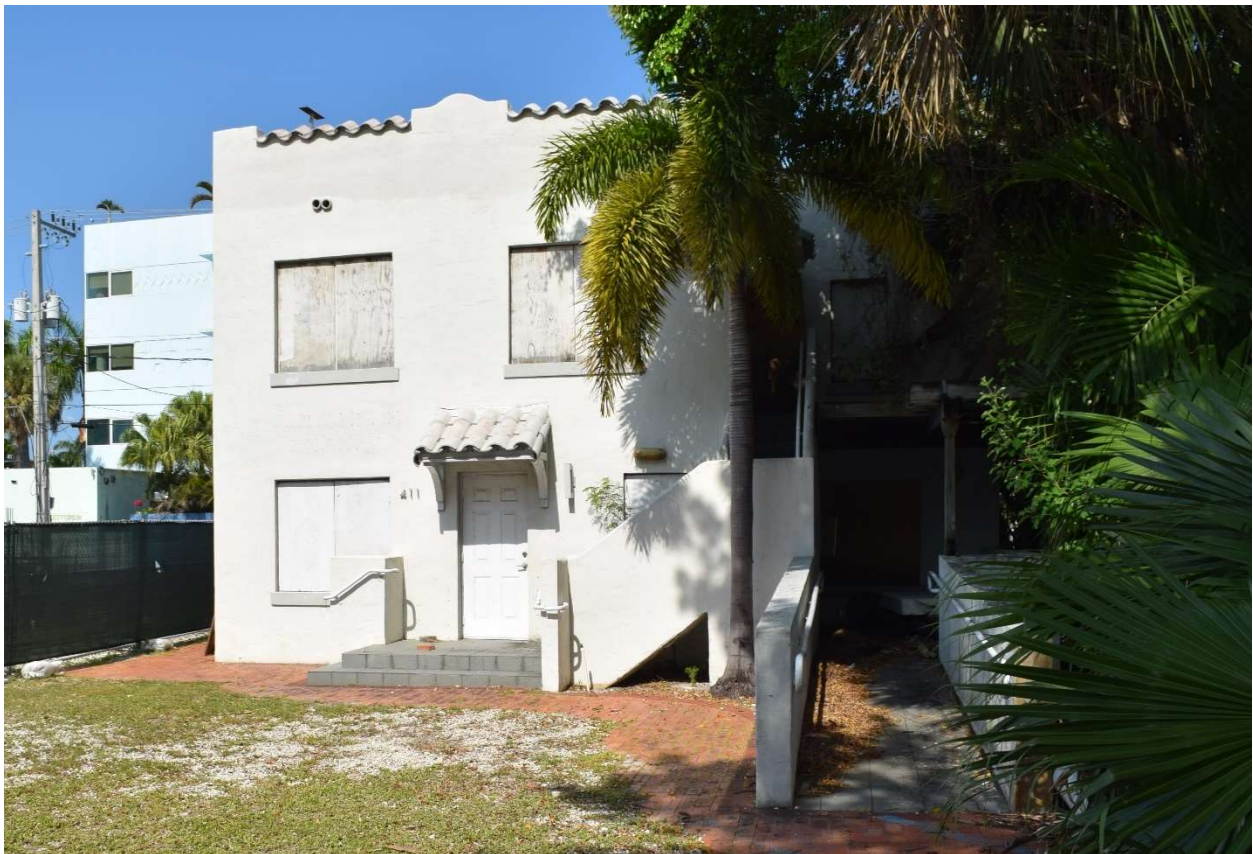
Fig. 15. Front façade of primary historic structure at 411 Michigan Avenue, May 2021.
