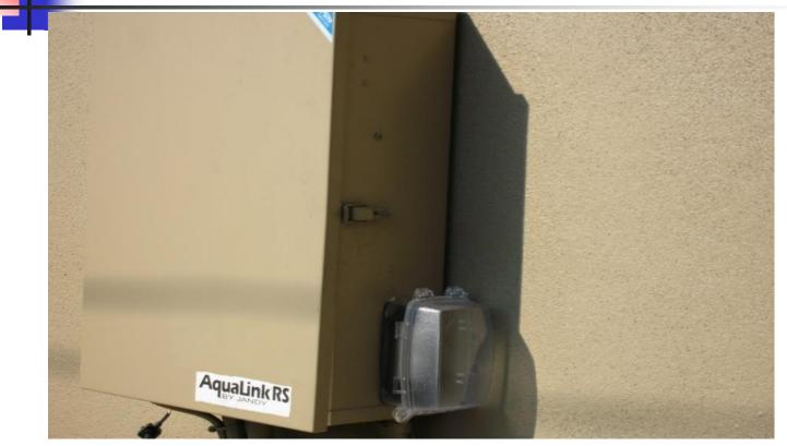
Check for GFCI receptacle minimum of 10' and maximum of 20' from water's edge
