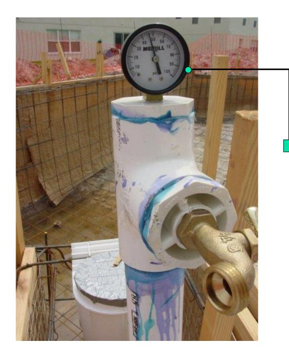
Pressure Rig **Pressure** test at 35#,s for 15 minutes. Or static test R4501.12 Tests section R4501.12.1
