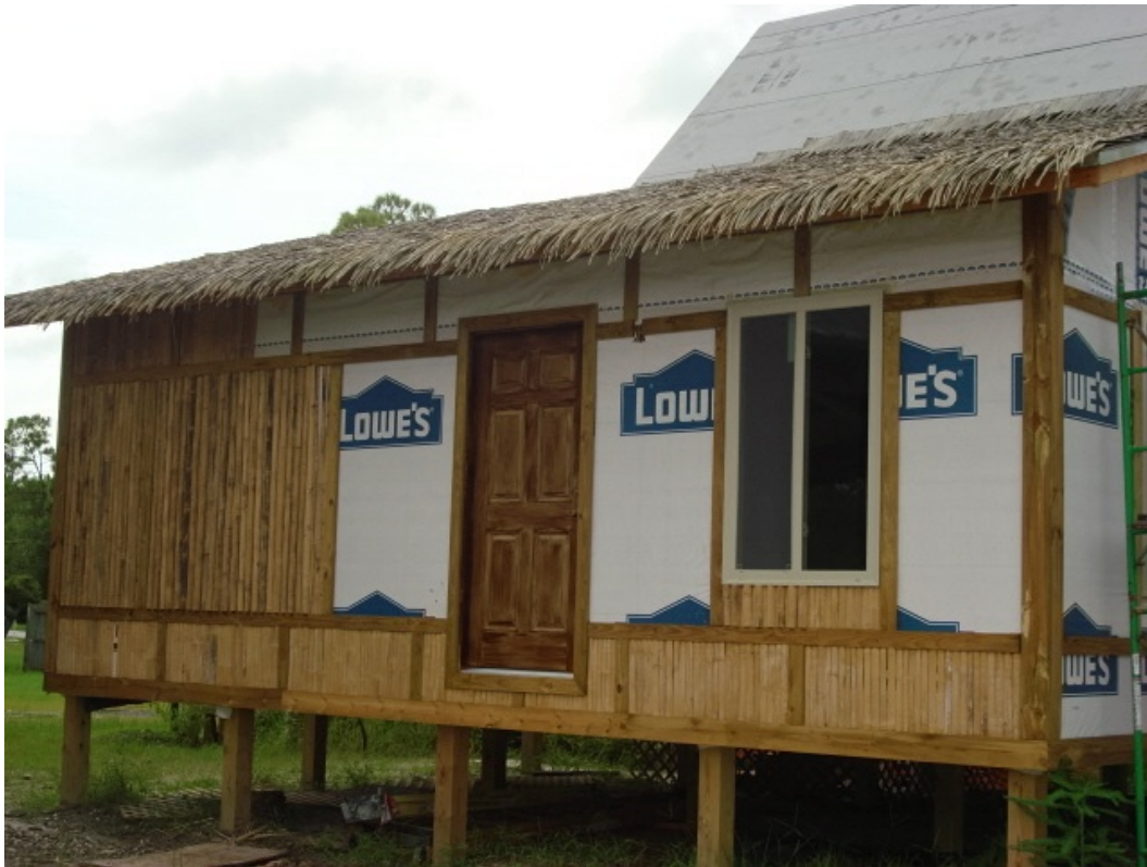
EAST SIDE - BAMBOO SIDING INSTALLATION IN PROGRESS
