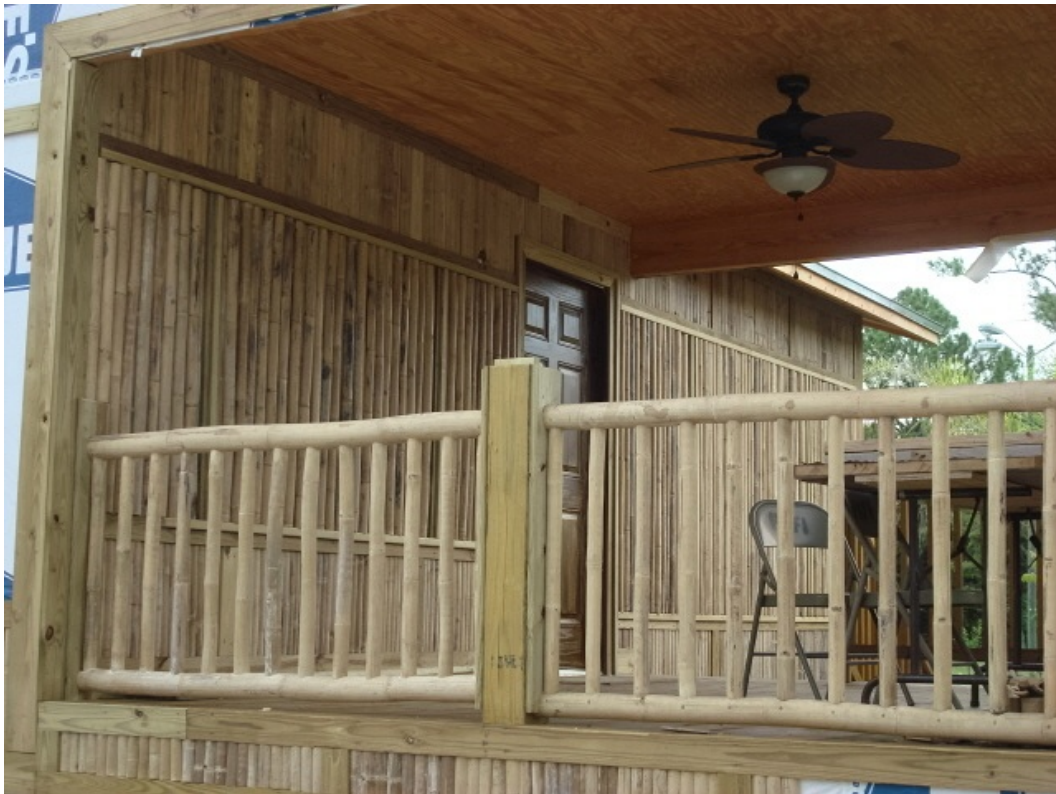
CLOSE UP OF BAMBOO RAILING AND SIDING
