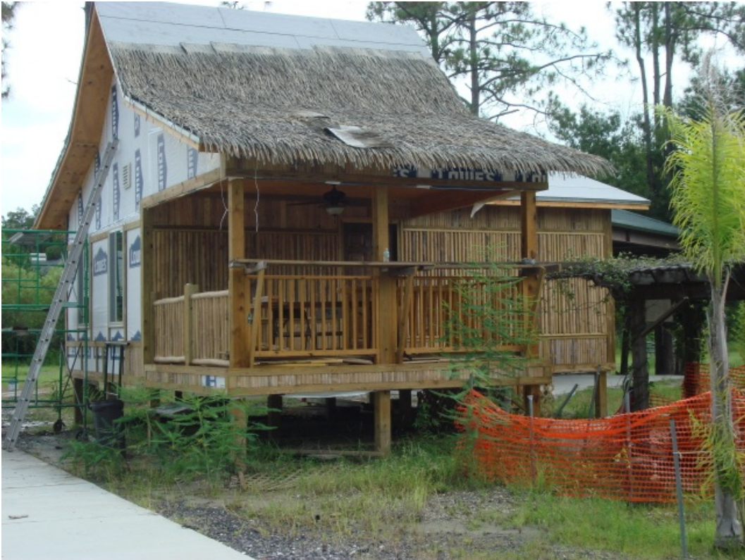
WEST SIDE - THATCH ROOF AND BAMBOO SIDING INSTALLATION IN PROGRESS
