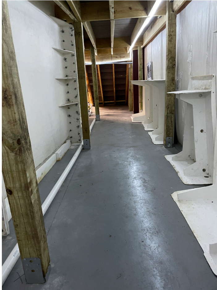
View down exterior building wall toward stairs
