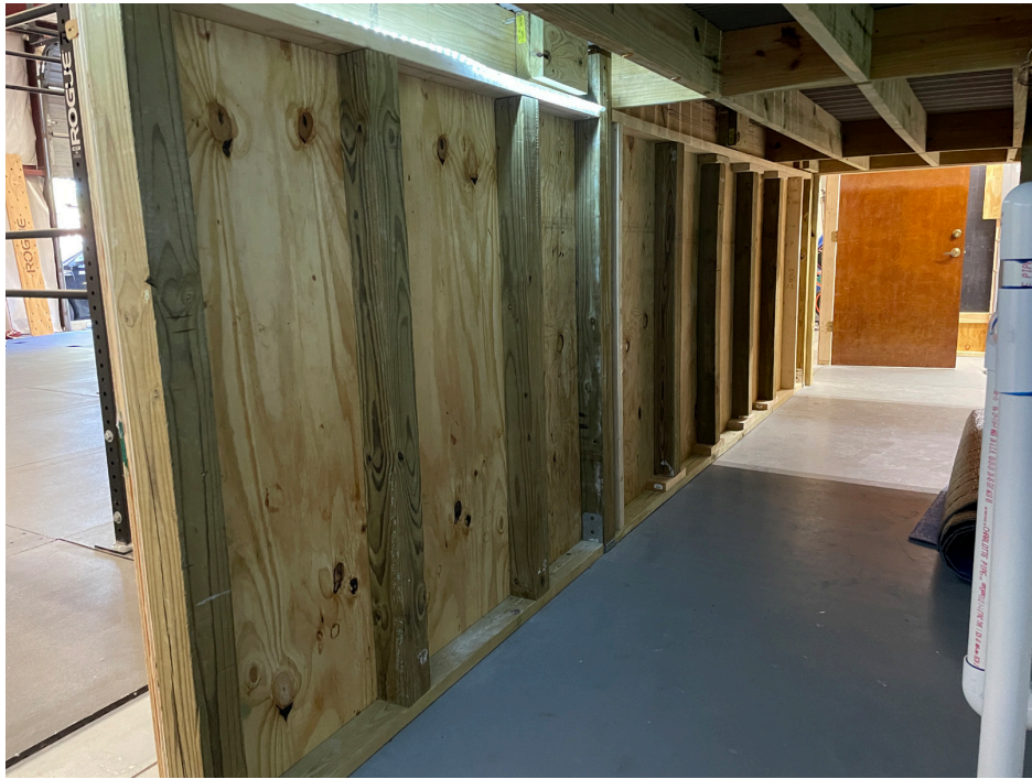
View down exterior deck wall toward pump room from sliding door
