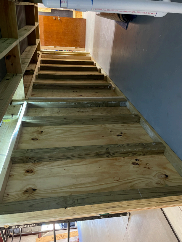
Wall E (view from inside sliding door toward pump room)
