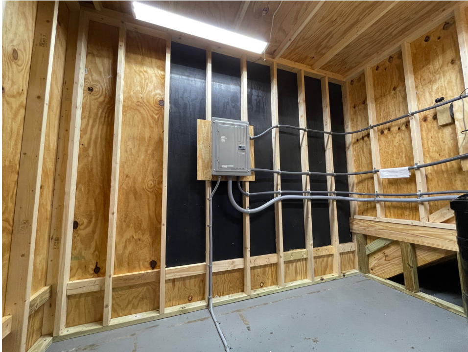
Wall D (view from inside pump room)
