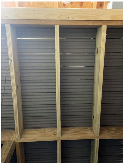
View of deck joists from below
