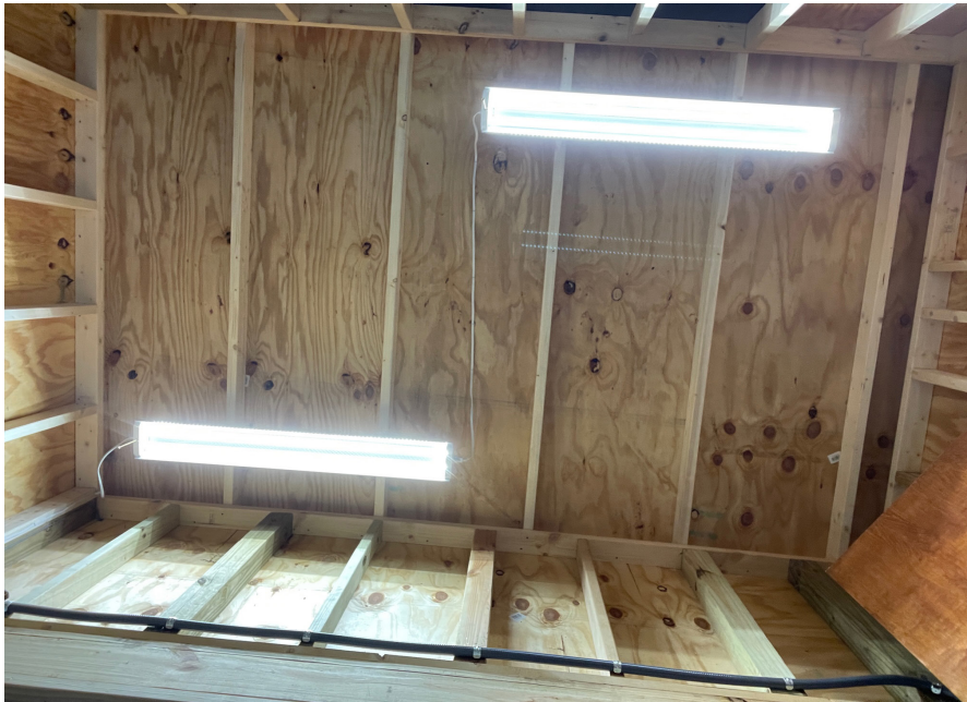
Pump room ceiling
