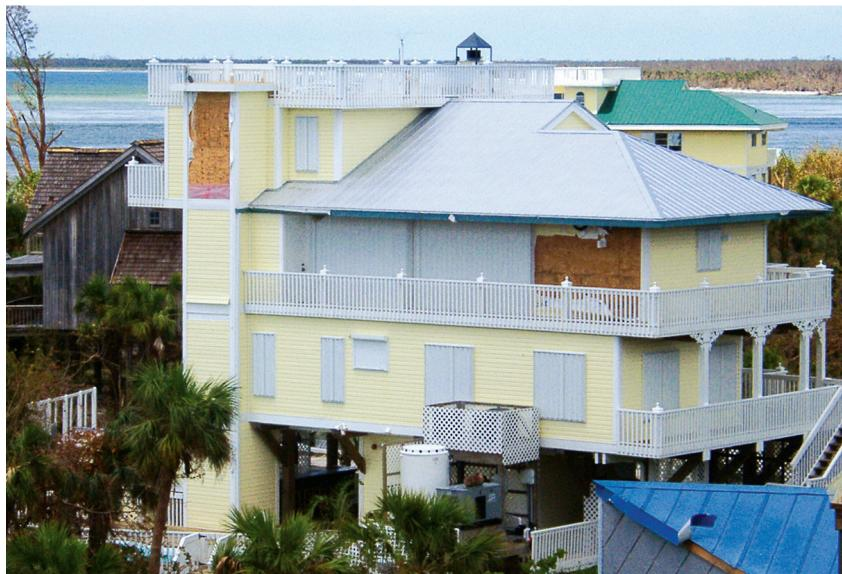
After Hurricane Charley, FEMA noted no structural damage to new wood-frame buildings built to the 2001 Florida Building Code standards.
