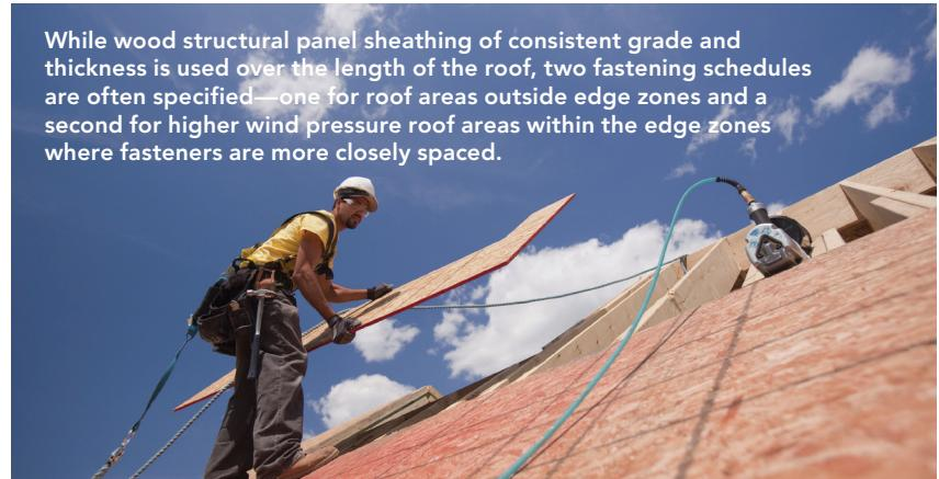
While wood structural panel sheathing of consistent grade and thickness is used over the length of the roof, two fastening schedules are often specified—one for roof areas outside edge zones and a second for higher wind pressure roof areas within the edge zones where fasteners are more closely spaced.
