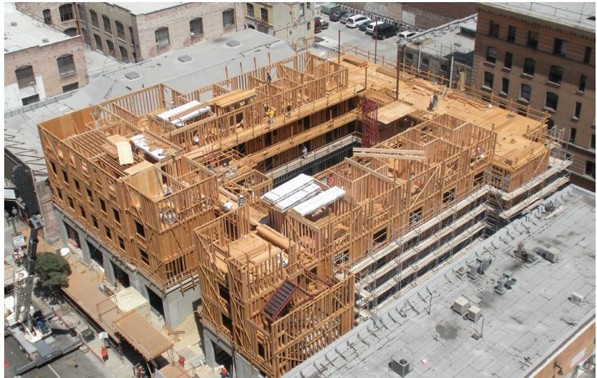
**Wood buildings are often characterized by repetitive framing and numerous connections—which provide multiple, often redundant load paths for resistance to wind forces.**
