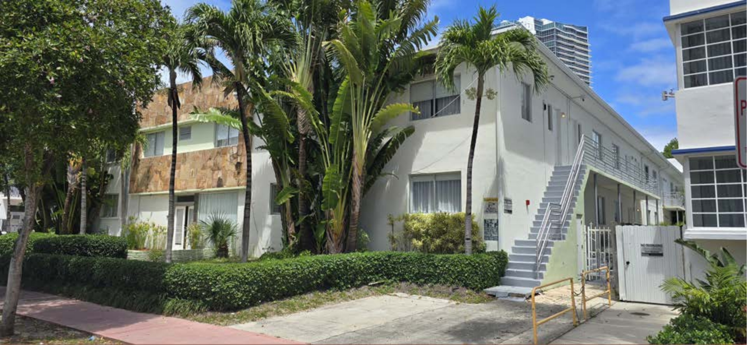
Southwest corner of Property – looking North from James Ave
