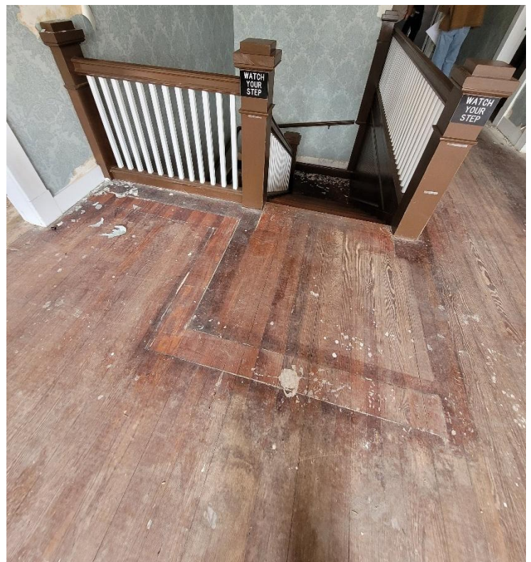
Stair Landing at Second Floor
