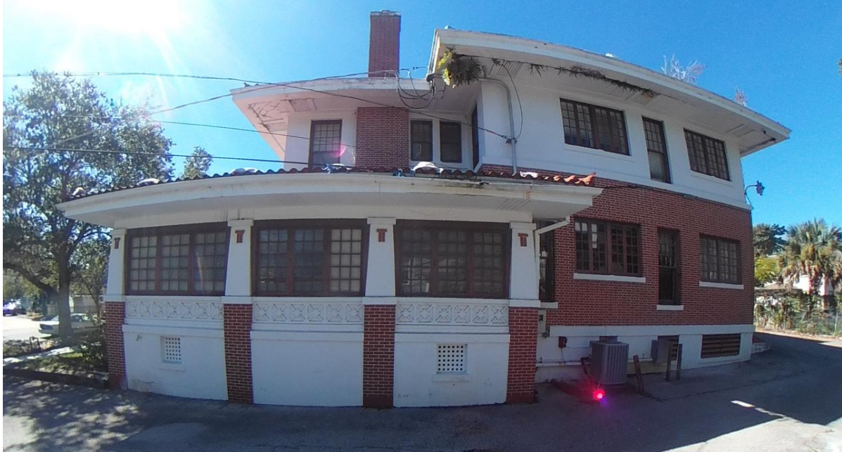
Existing Building - Right Side
