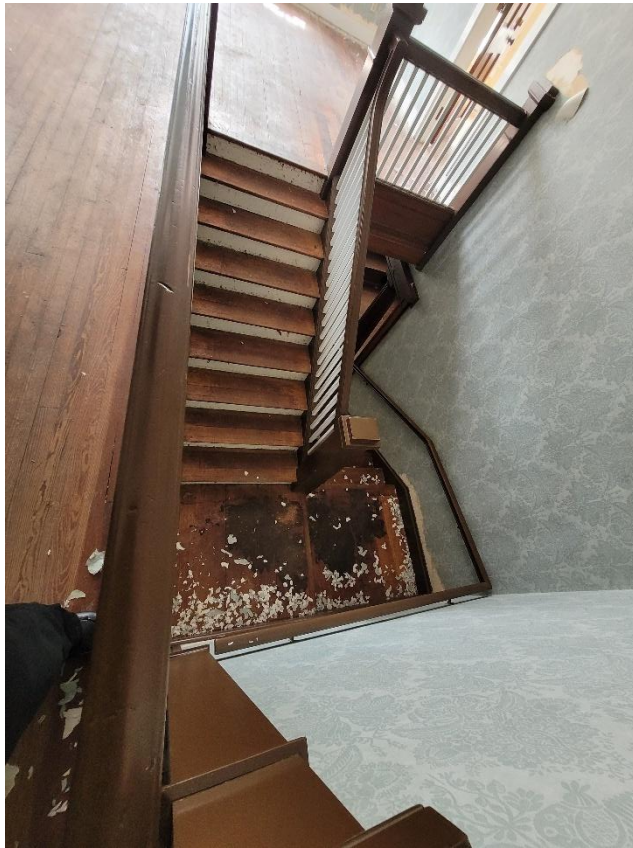
Stair to Second Floor
