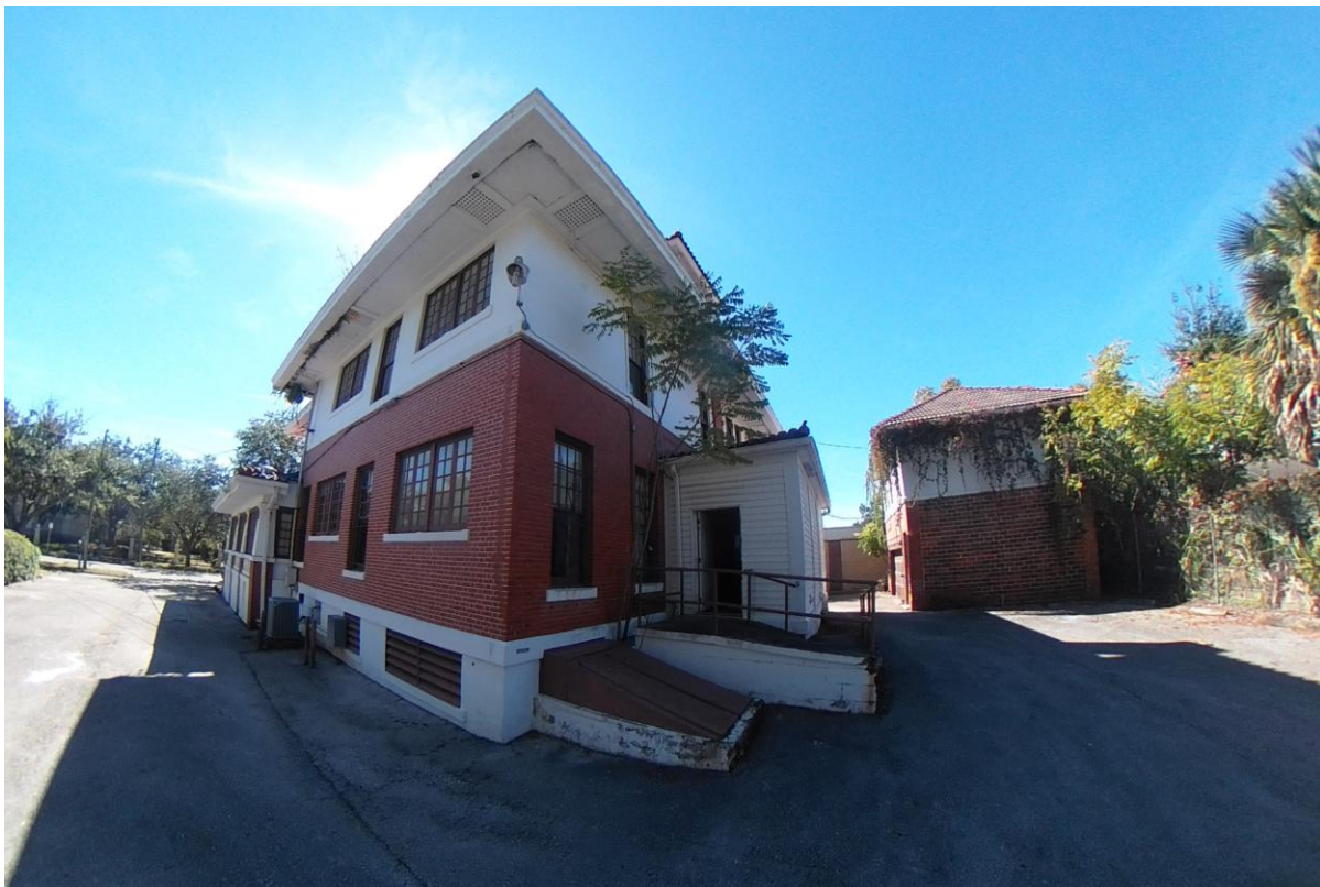
Existing Building - Partial Right Side & Rear Side, Right side of Garage
