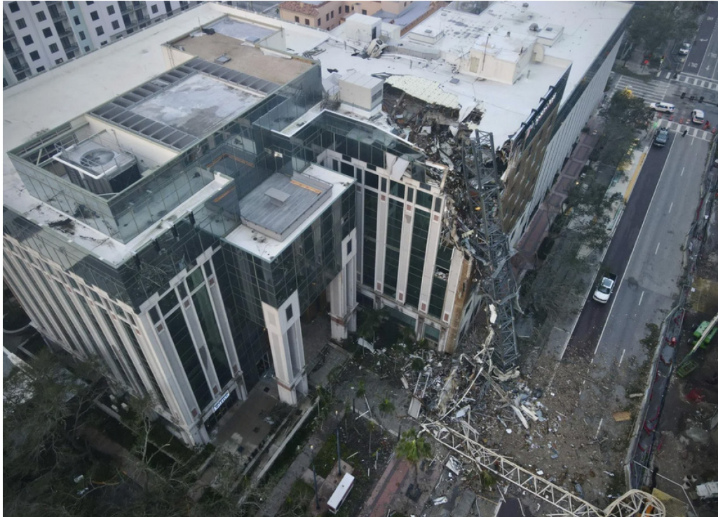
Figure 4-9. Tower crane collapsed into building in St. Petersburg, Florida. [25]
