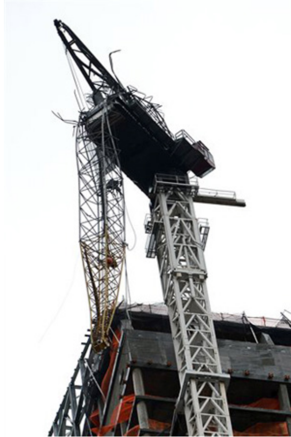
Figure 4-5. Tower crane destroyed during Hurricane Sandy in New York City. [20]
