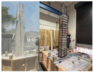
Figure 24. Column Sandblasting and Shell Retrofit
