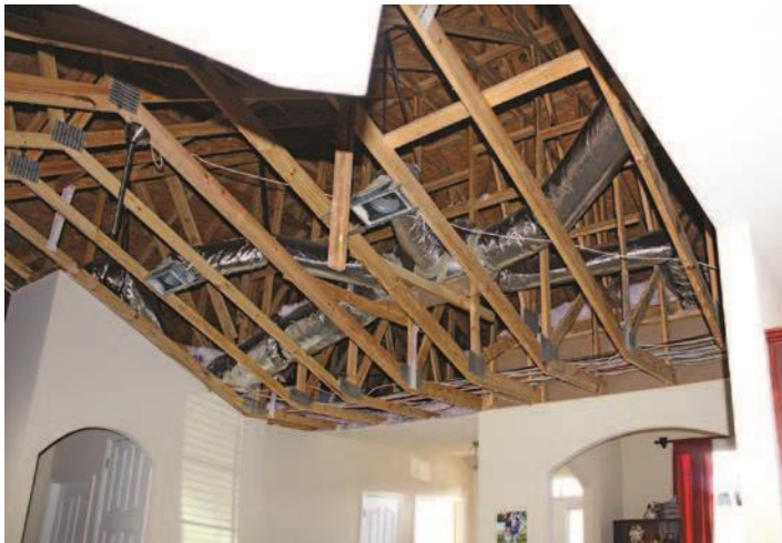
Figure 1: House with significant interior damage from water intrusion (FEMA, 2019)
