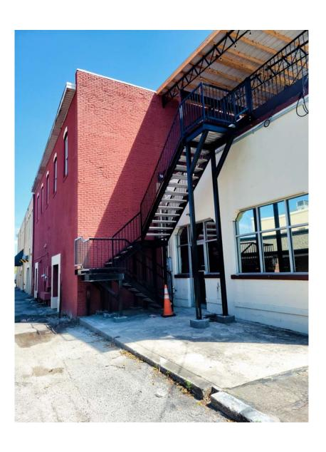
This is the north side of the building where we installed the emergency egress staircase. The front corner is where the electric power lines are attached to the building from the service pole.
