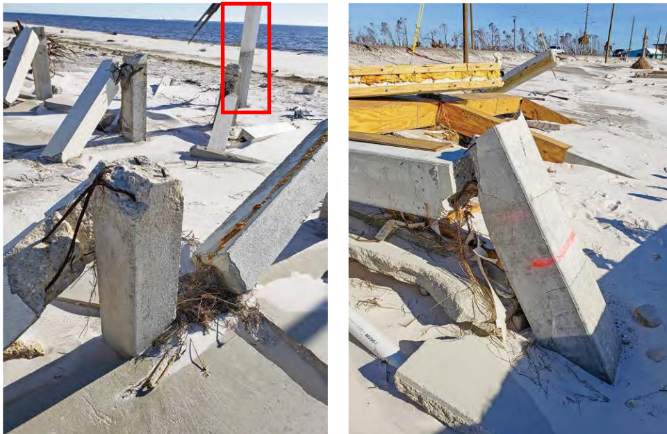
Figure 1. Examples of failed concrete piles during Hurricane Michael (adapted from FEMA [1]). Note that the pile closest to the shoreline (pile boxed in red) did not fail.
